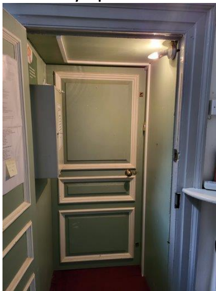
Inside of key cupboard on first floor
