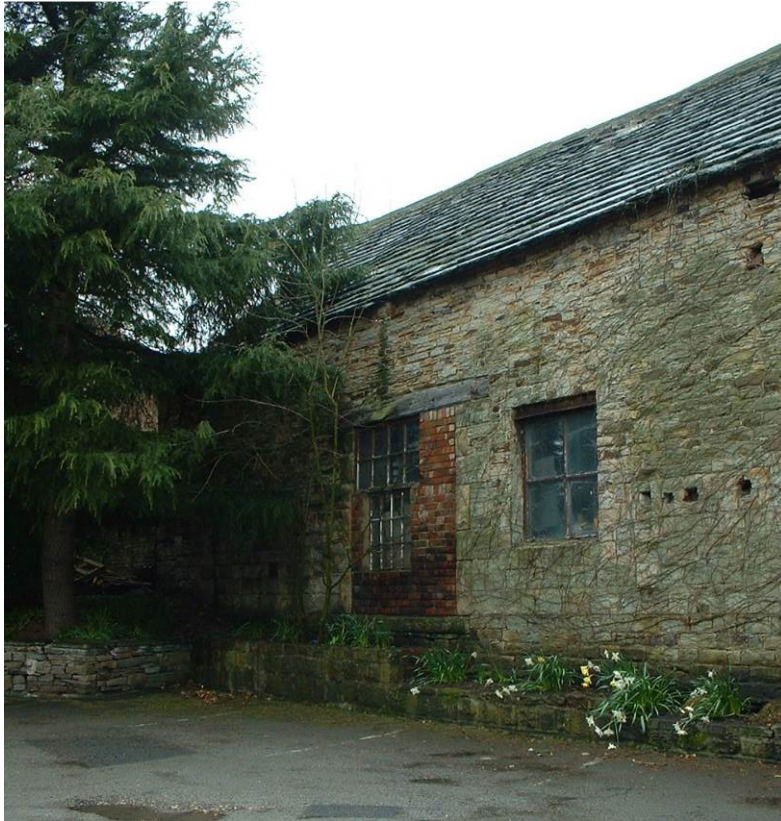
05. Rear wall of barn – North East Elevation.
