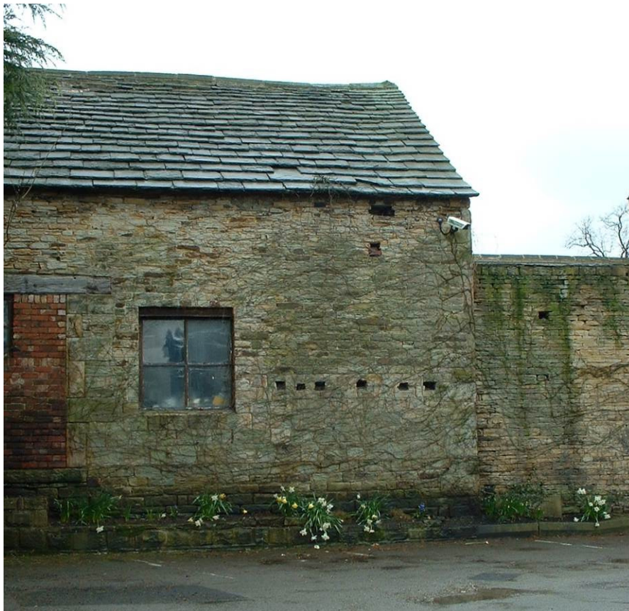
06. Rear Wall of barn – North East Elevation
