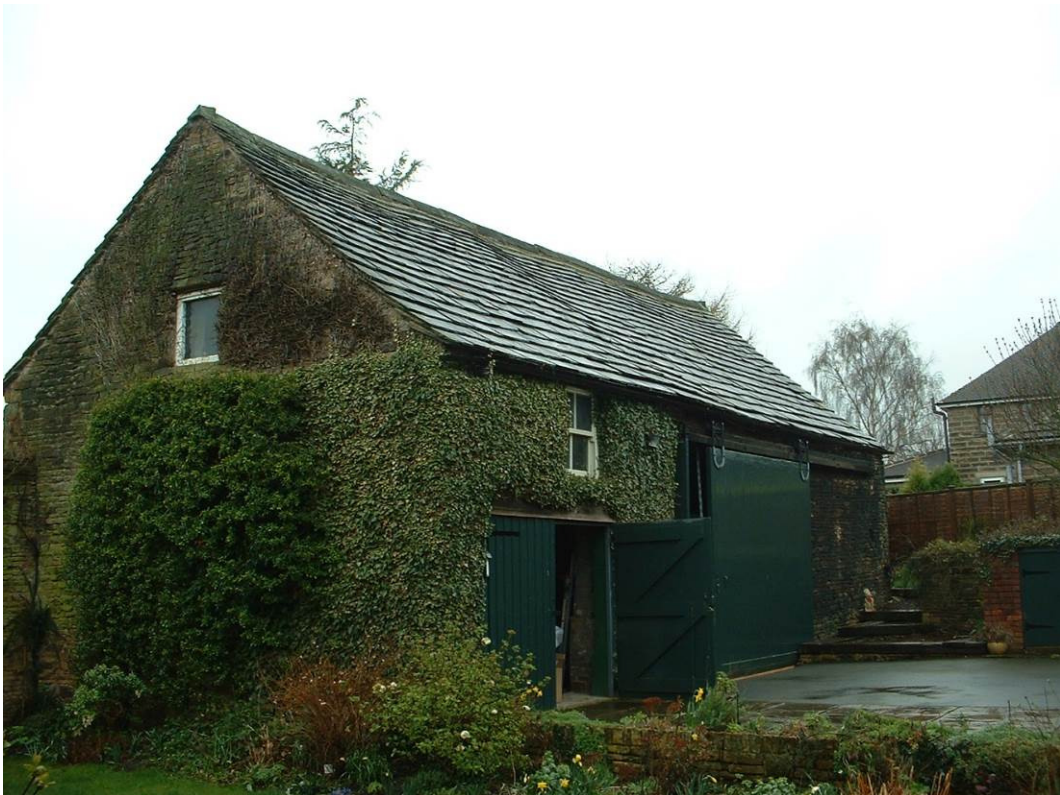
04. North East and North West Elevation taken before ivy removal.
