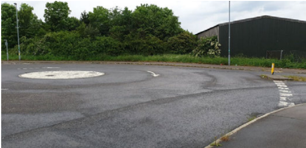
Figure 19 - View from eastern leg to northern leg.
