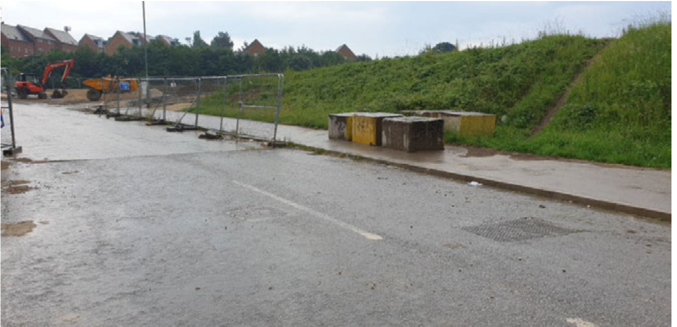
Figure 27 - View of existing footway alongside S38 section of works.
