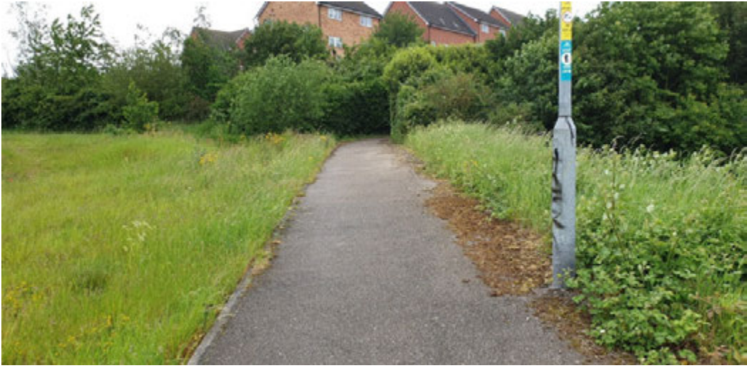
Figure 49 - Footway in good condition toward link through to beyond site boundary.
