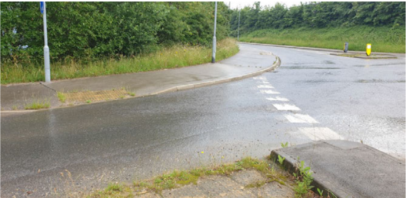
Figure 34 - View across northern island to eastern side.
