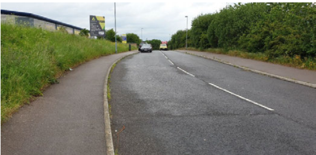
Figure 8 - Southern footway on Ashroyd Way looking west.
