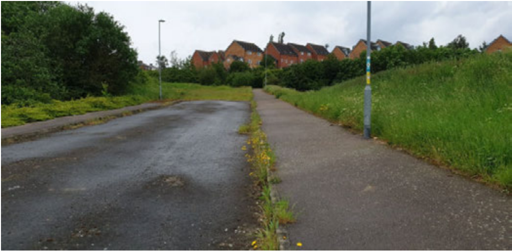
Figure 42 - Western channel looking south.
