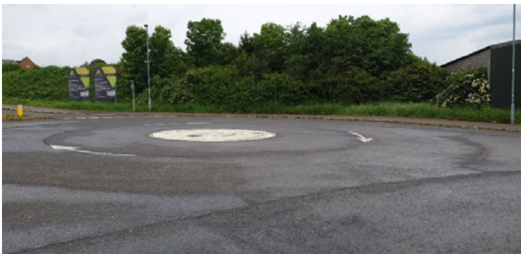
Figure 20 - View of surfacing across mini roundabout.
