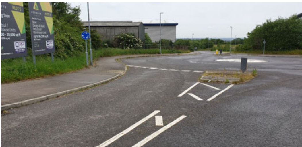
Figure 26 - Approach to roundabout on southern leg.
