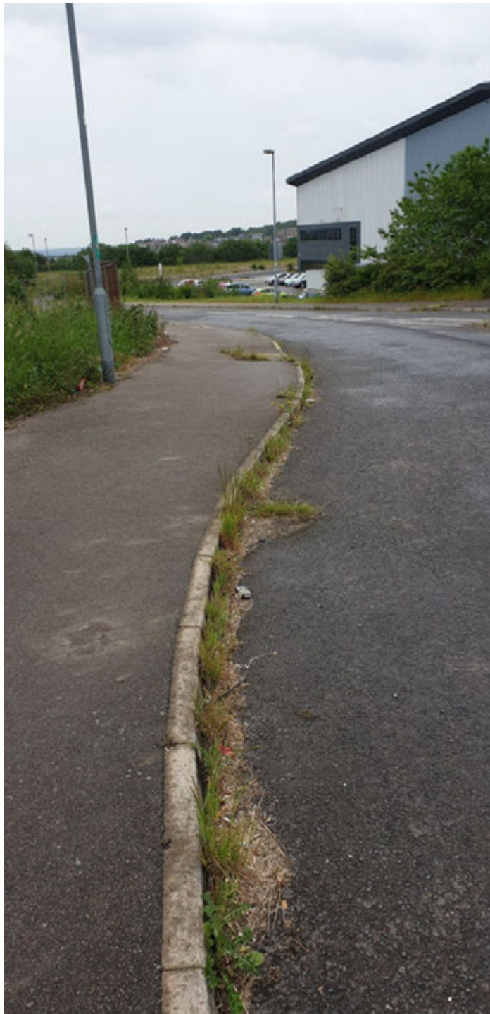
Figure 29 - Kerb line on western side of roundabout looking toward the northern leg.
