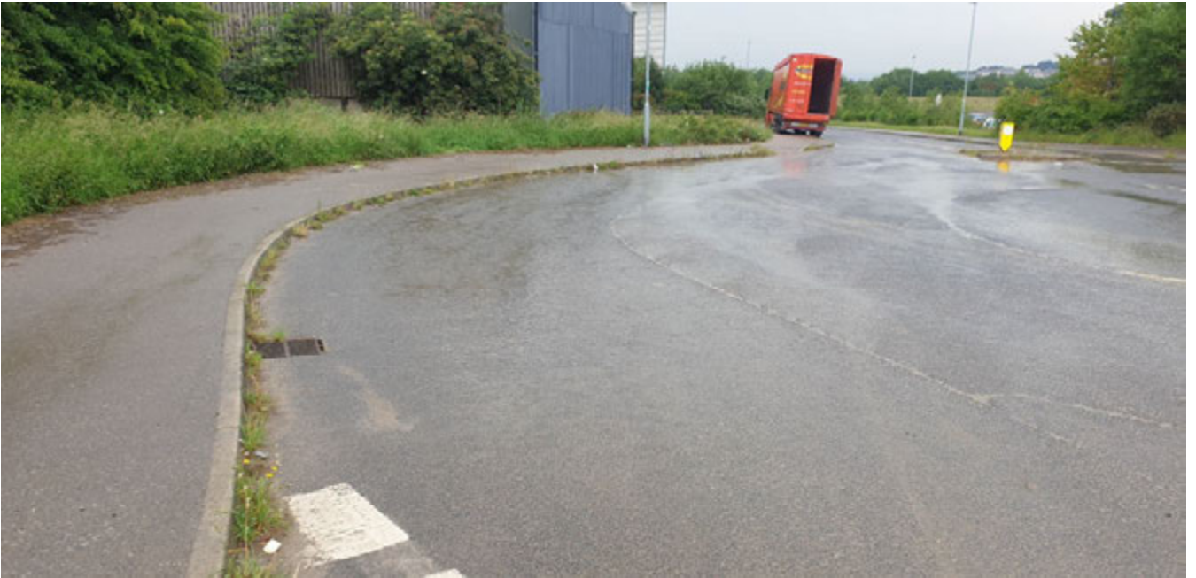
Figure 31 - View of western side of roundabout - vegetation within channel line.
