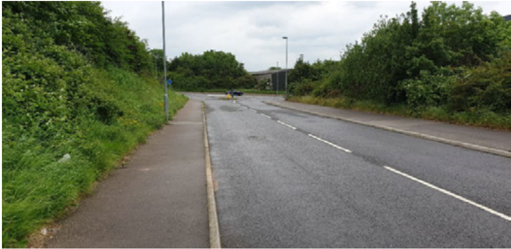
Figure 15 - View west on approach to mini roundabout.
