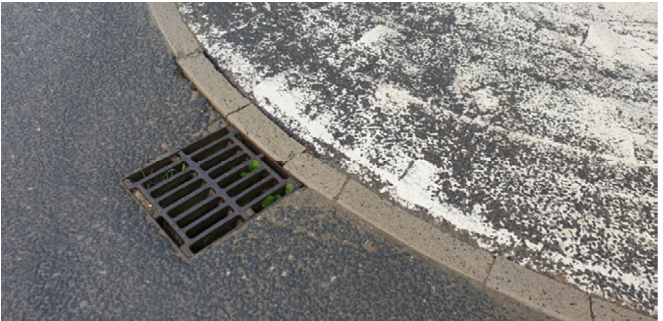
Figure 21 - View of centre island at roundabout. Note the damaged kerb next to the gully was present prior to works starting at was noted on the pre-start report.
