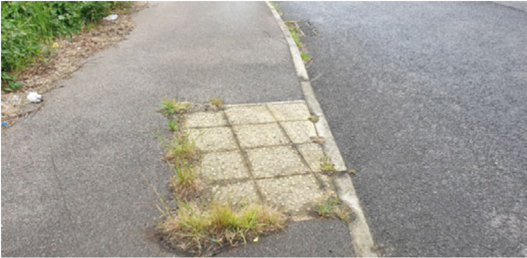
Figure 30 - West side of northern leg - tactile pavers.
