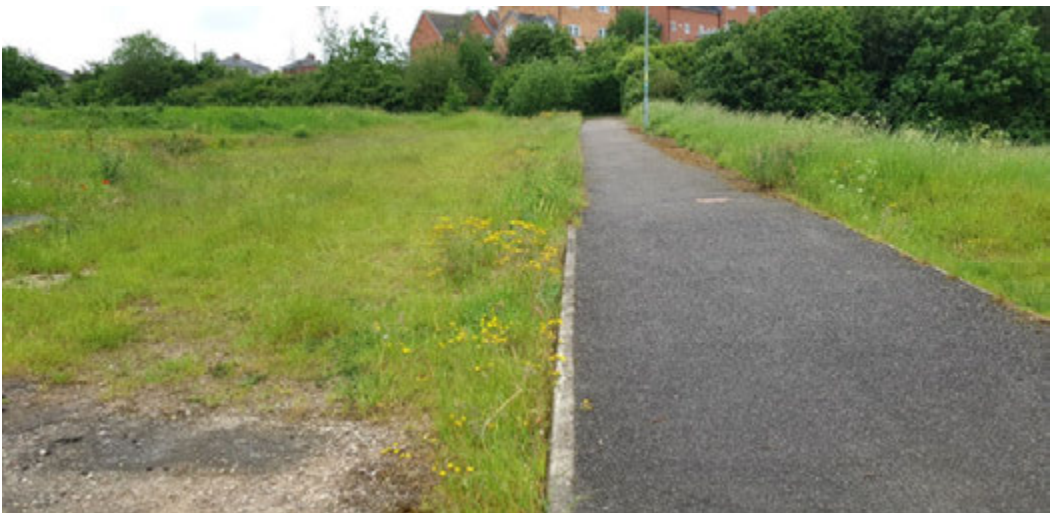
Figure 48 - Footway continuing south toward end of site boundary. Footway in good condition. Carriageway incomplete.
