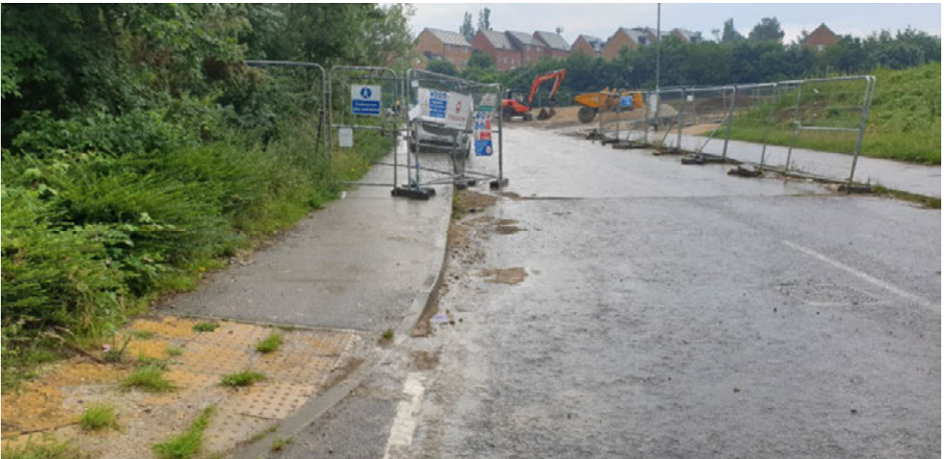
Figure 26 - View south into S38 section. Refer to Figure 45 Appendix B.
