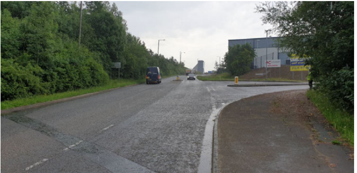
Figure 1 - View of north on Ryecroft Bank to junction with Ashroyds Way.
