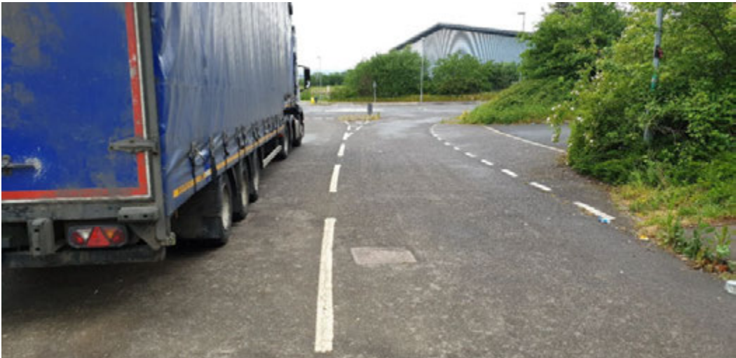
Figure 40 - Looking south - eastern side tactiles heavily overgrown, vegetation over footway.
