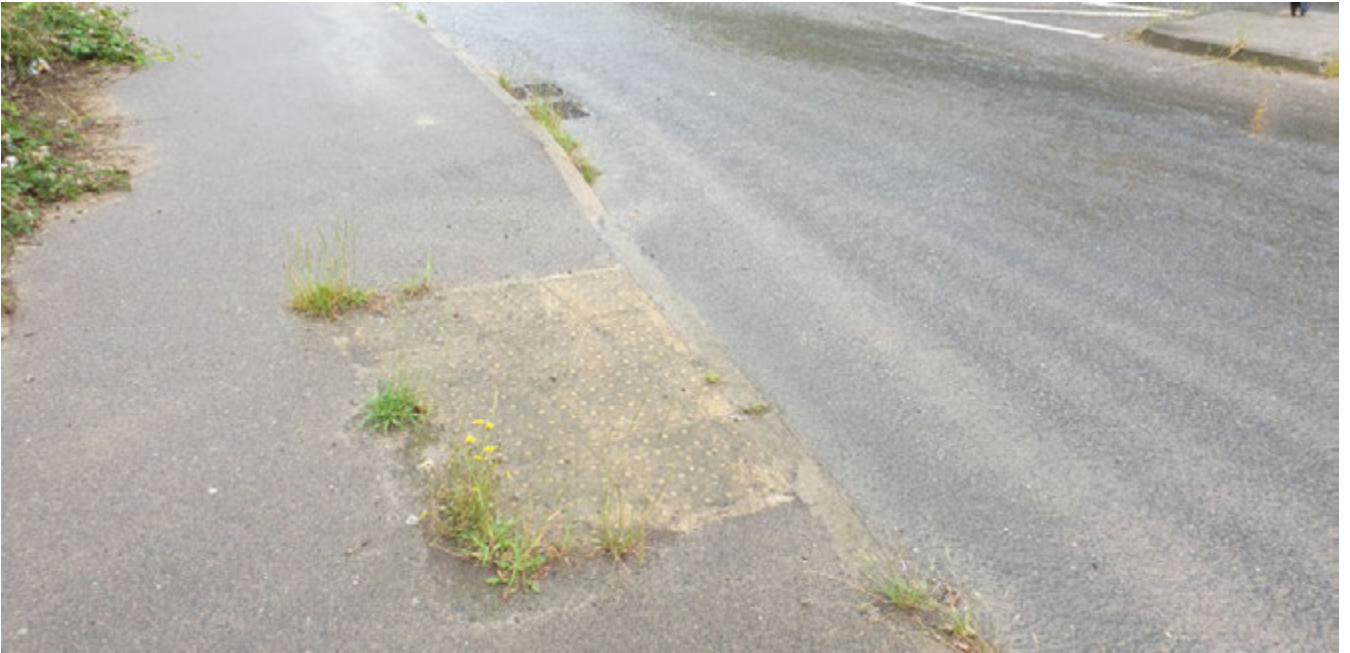
Figure 33 - View of tactile pavers on west side of southern leg.
