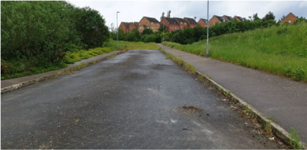
Figure 39 - View south beyond concrete blocks. Footway on western side is complete and surfaced. Carriageway is incomplete.
