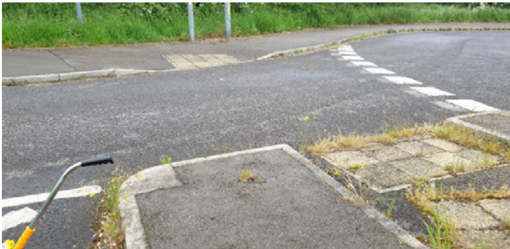
Figure 25 - Missing reflective bollard on southern side of island on southern leg.
