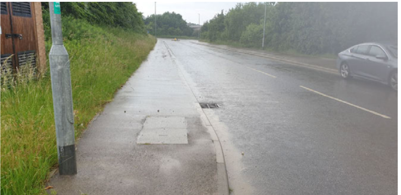
Figure 10 - View of footway in front of Storefirst (Plot 4A)
