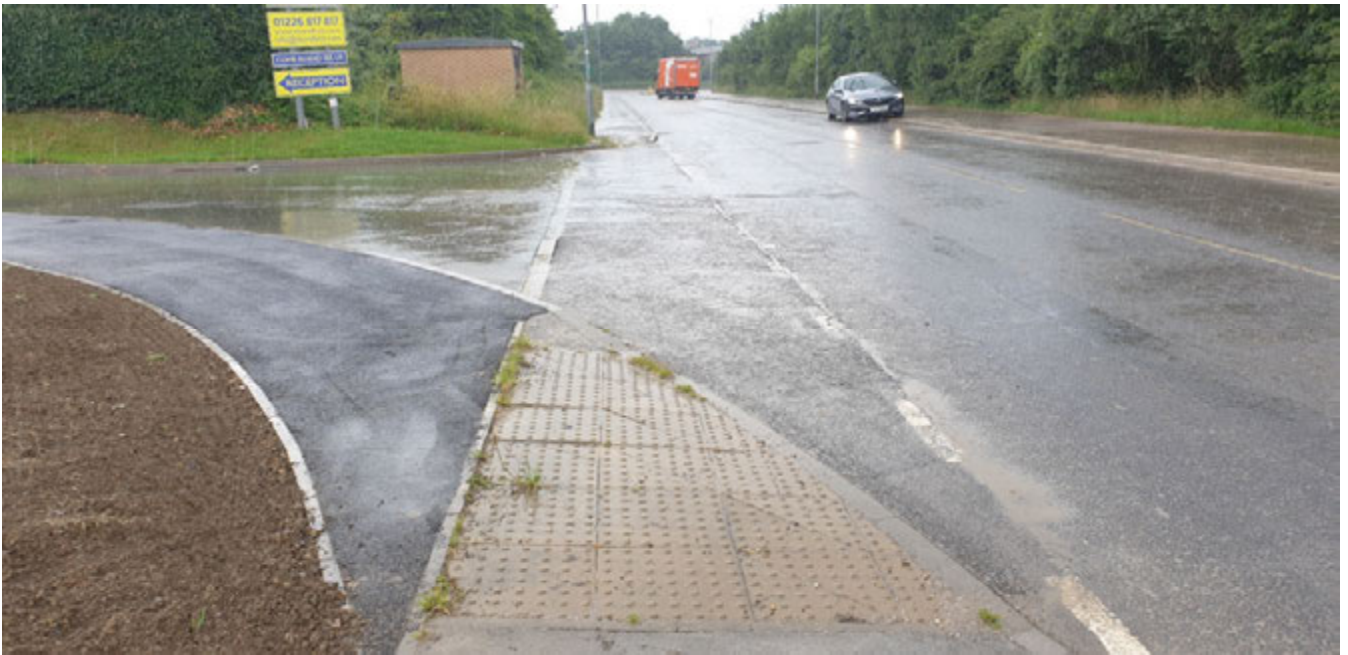
Figure 7 - View across Plot 4B entrance.
