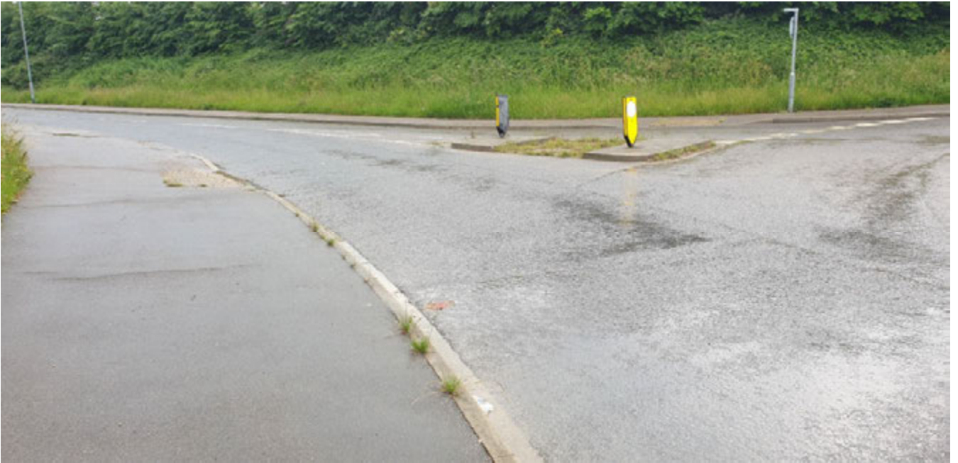
Figure 35 - View of Ashroyd Way (eastern leg from roundabout)
