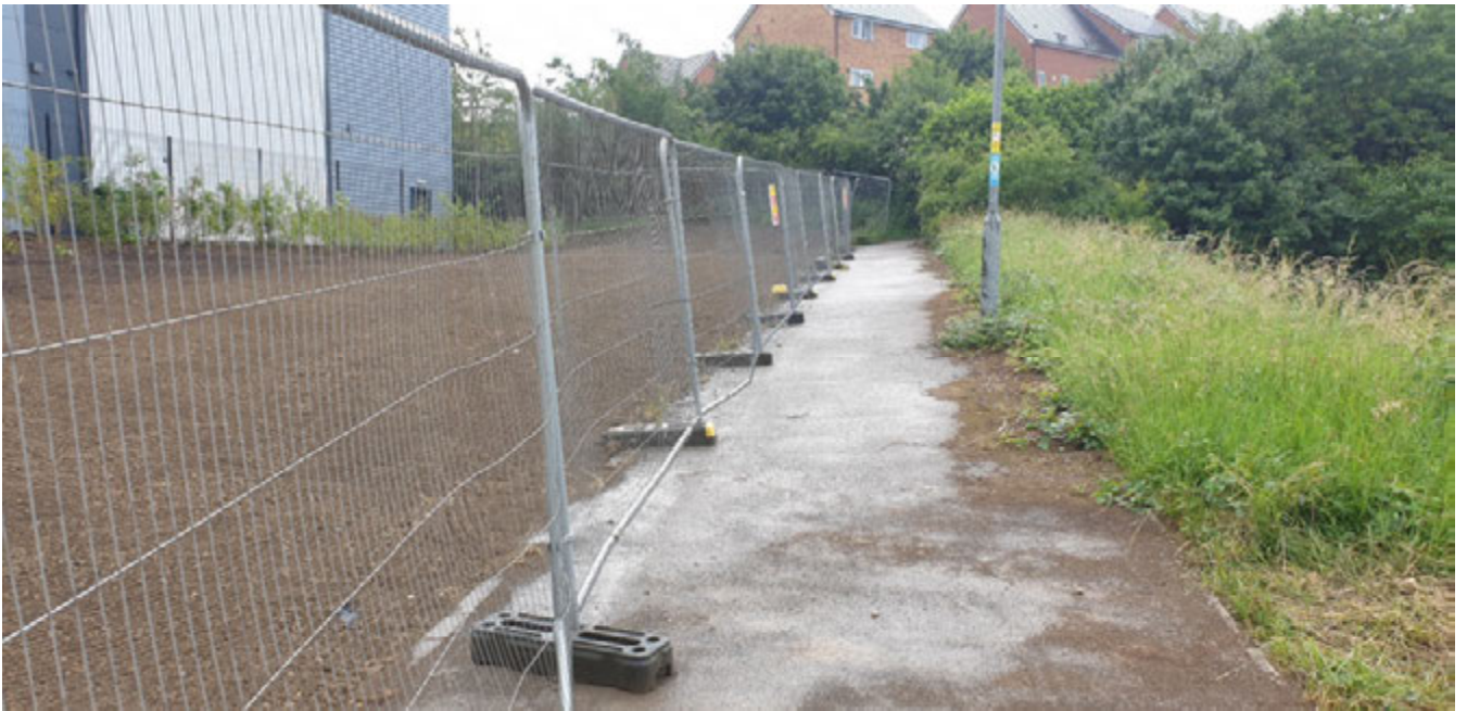
Figure 29 - Existing public footpath adjacent S38 area.
