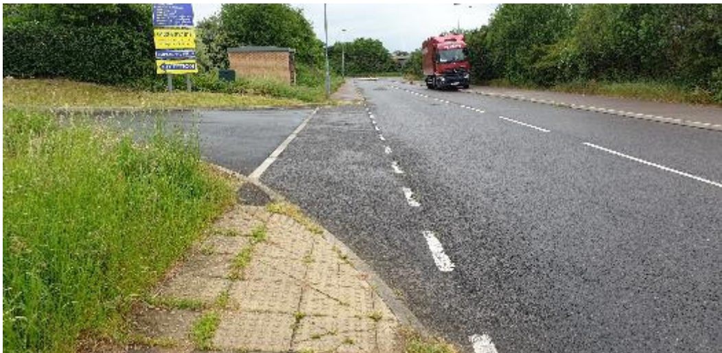
Figure 10 - View across entrance to Self-Store site/ Plot 4B entrance. Vegetation in tactile pavers.
