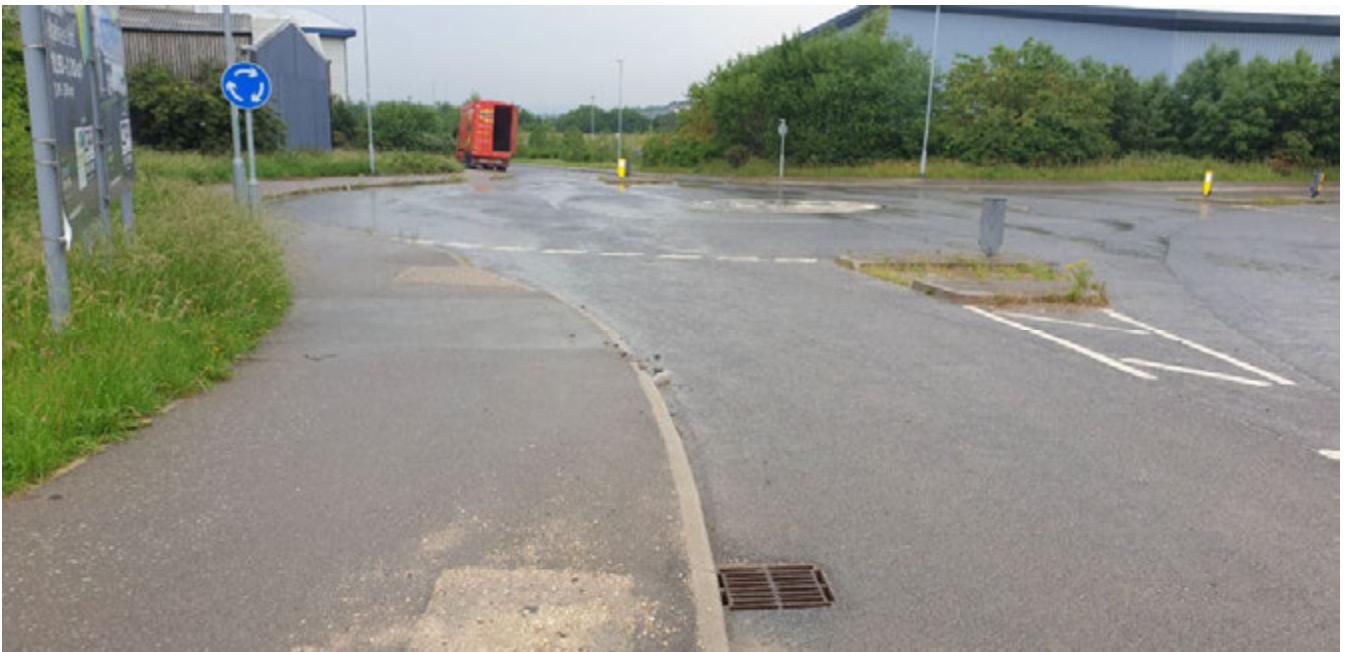
Figure 30 - View north from southern leg, bollard on island was missing prior to works commencing.
