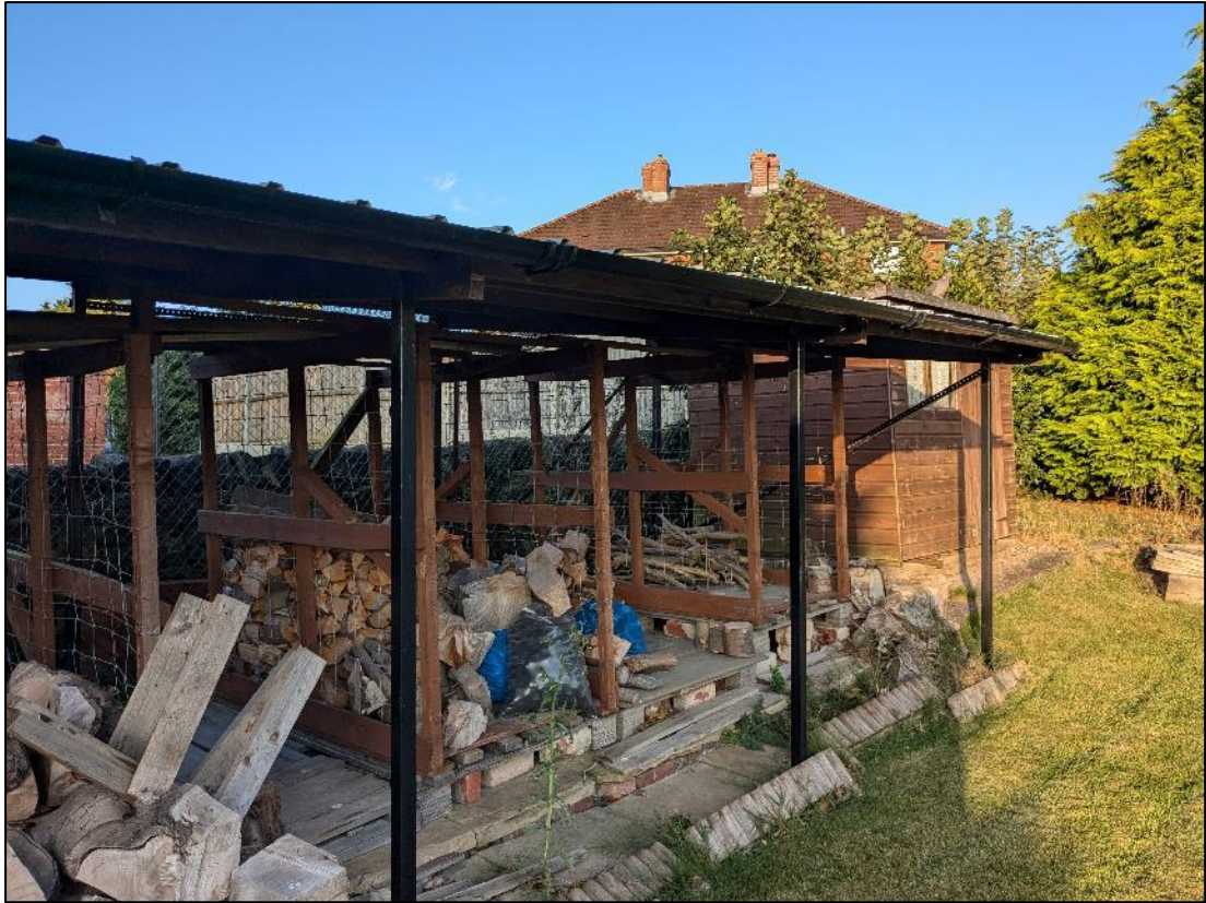
Plate 7. Southwest elevation of B2 & B3
