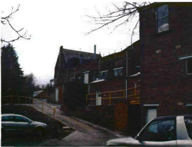
View looking North West of site showing existing access into the site from Saville Lane. Existing offices can be seen in the background.
