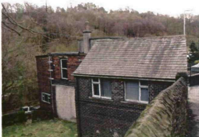
View along the South Eastern elevation of the Site showing rear of existing office buildings.
