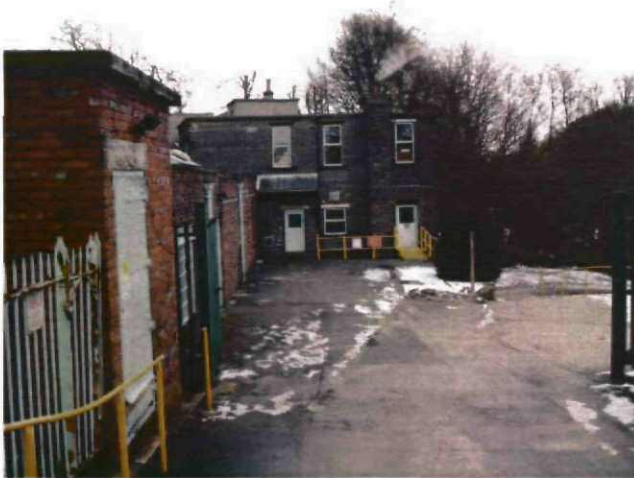
View North East of the site looking towards the existing office buildings to be demolished to form the base of the proposed office development.
