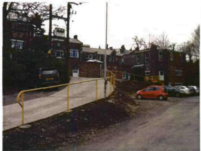
View North East of the site showing access to the South West of the site. Existing offices can be seen in the background.
