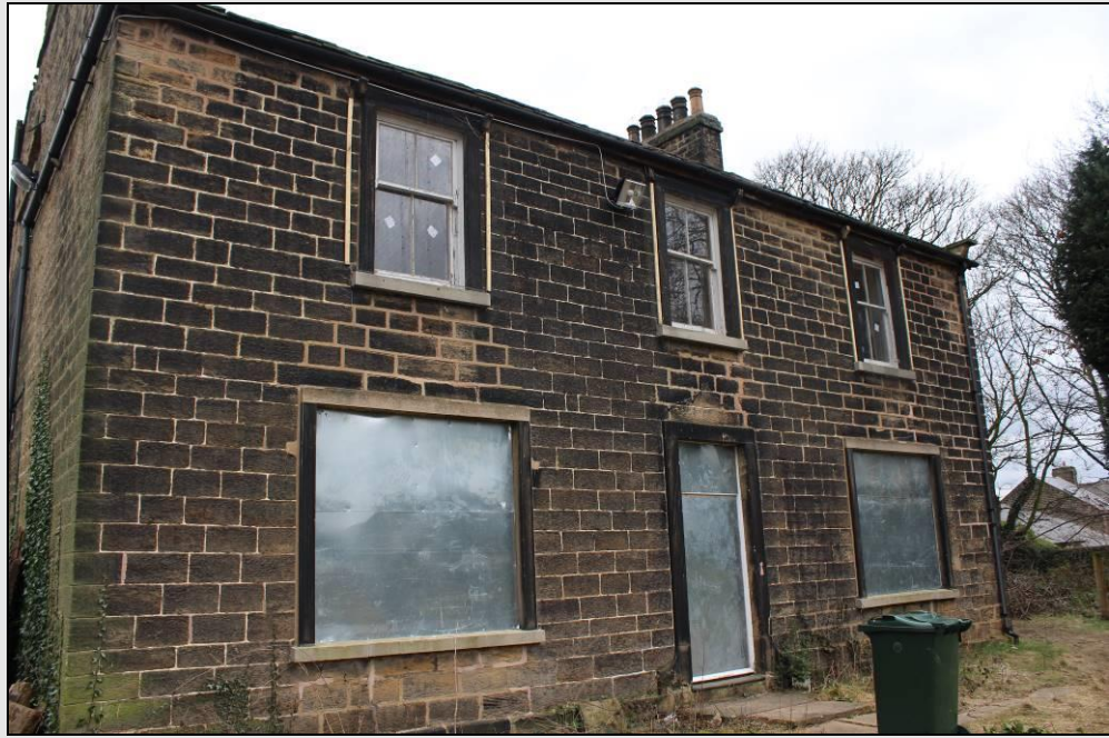
Figure 7. External view of the north-east face of Building 1A.
