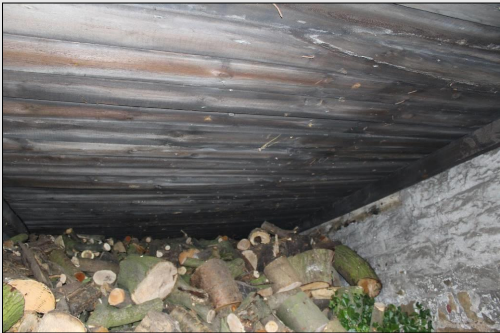
Figure 25. Internal view of Building 3A, showing tightly fit sarking.
