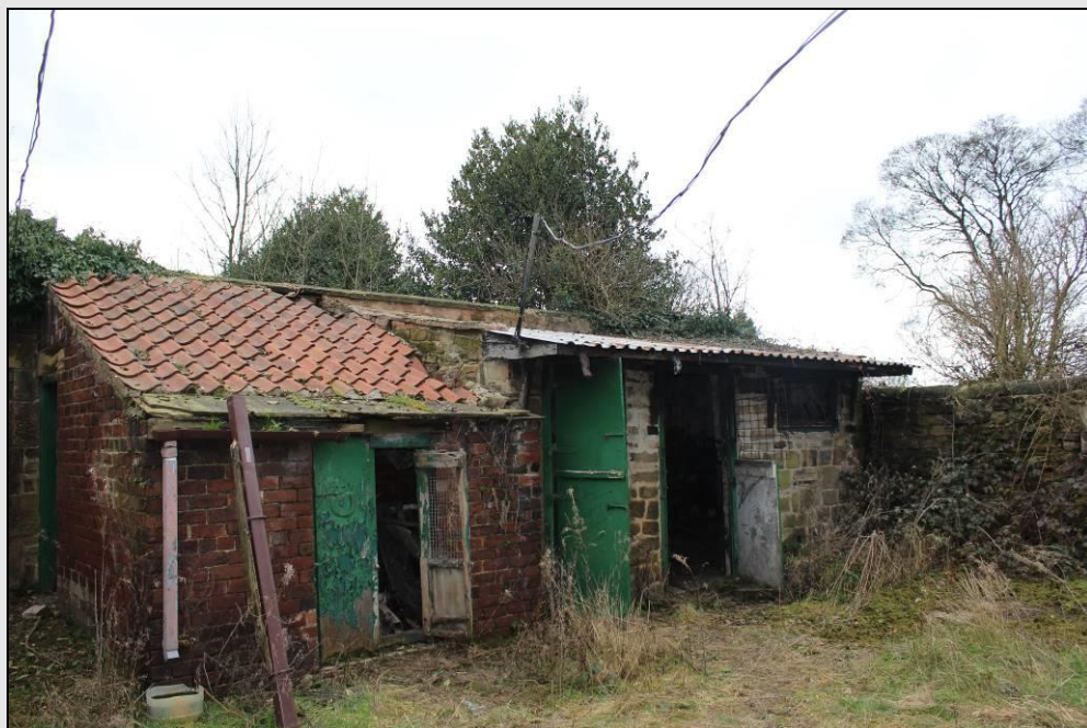
Figure 36. External view of the north-eastern face of Buildings 4A (right hand side) and 4B (left hand side).
