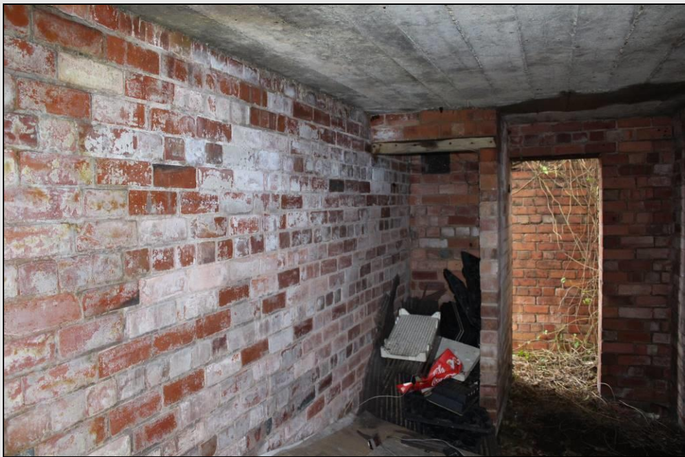
Figure 43. Internal view of Building 5, including entrance at north-eastern end.
