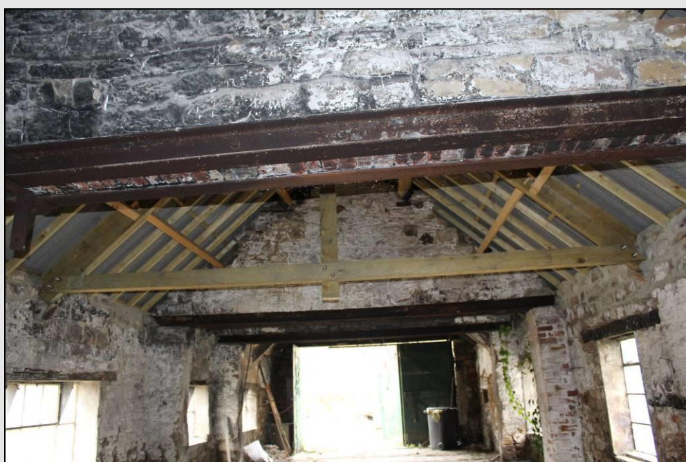
Figure 20. Internal view of Building 2, showing open doors at south-west end of building and new wooden beams supporting the roof.
