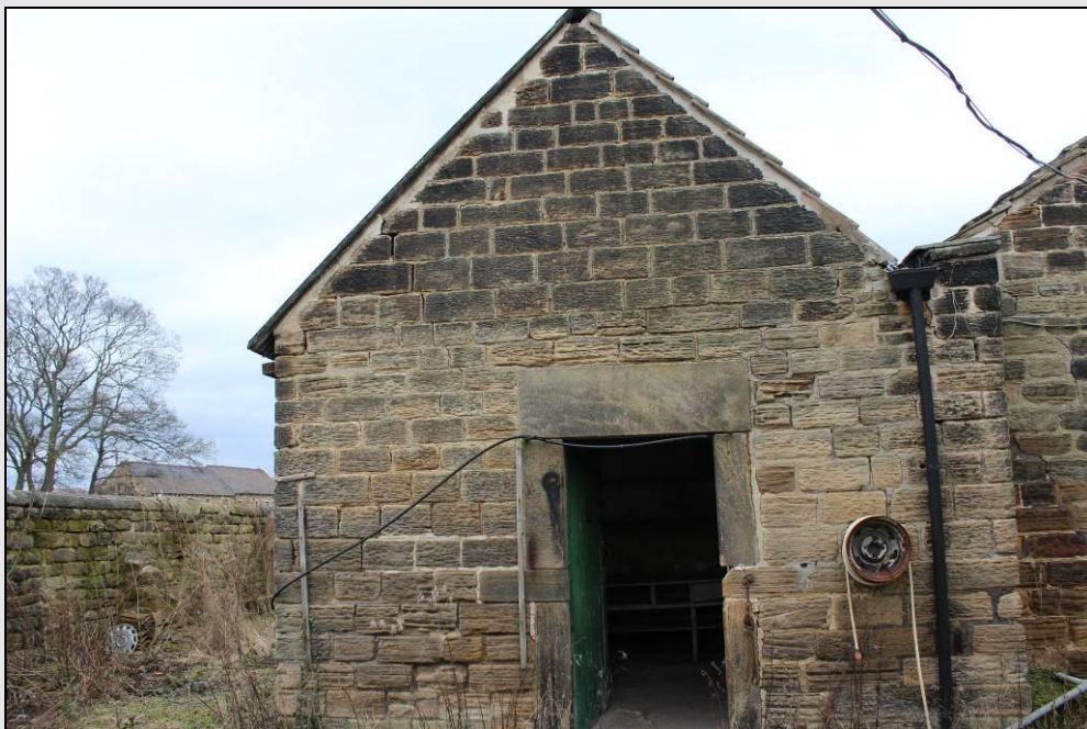
Figure 27. External view of the south-west face of Building 3B.
