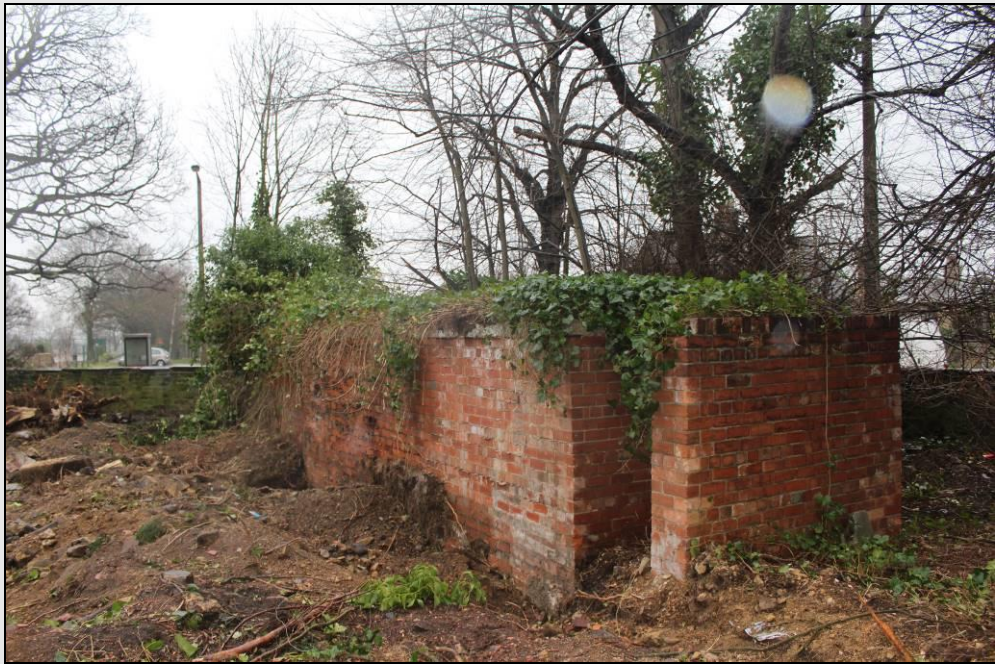
Figure 42. External view of Building 5 from the western corner of the building, showing heavy ivy cover on roof of building.
