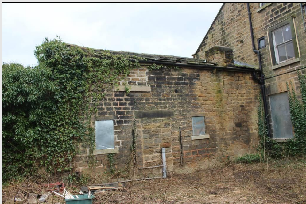
Figure 13. External view of south-west face of Building 1B.
