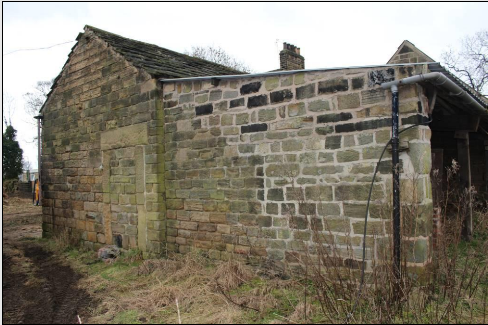
Figure 32. External view of north-east face of Building 3C (right hand side) and 3A (left hand side).
