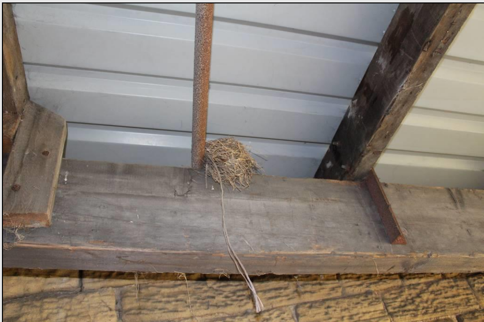
Figure 35. Internal view of Building 3C, showing disused bird's nest on wooden beam.
