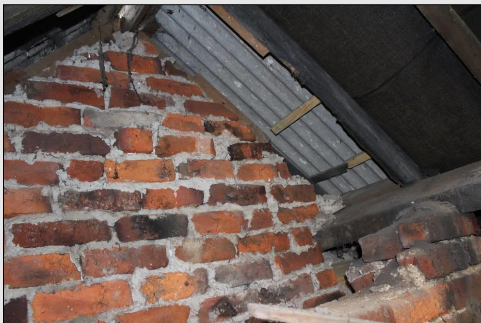
Figure 29. Internal view of loft space of Building 3B, showing potential entry point in the roof's apex.
