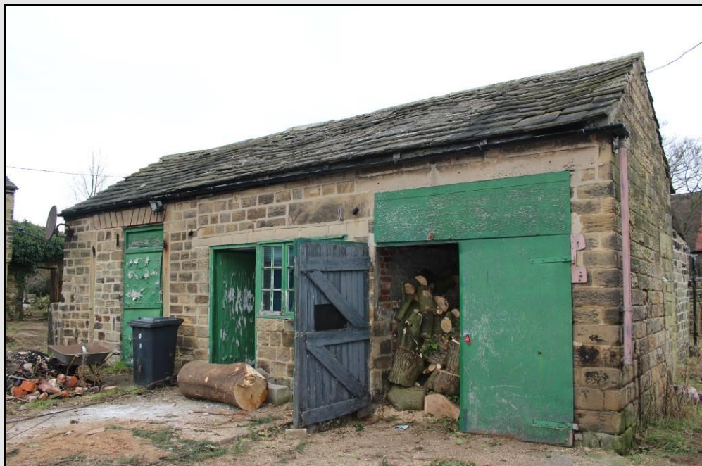
Figure 23. External view of the south-east face of Building 3A,
