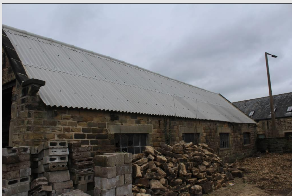
Figure 17. External view of the south-east face of Building 2.
