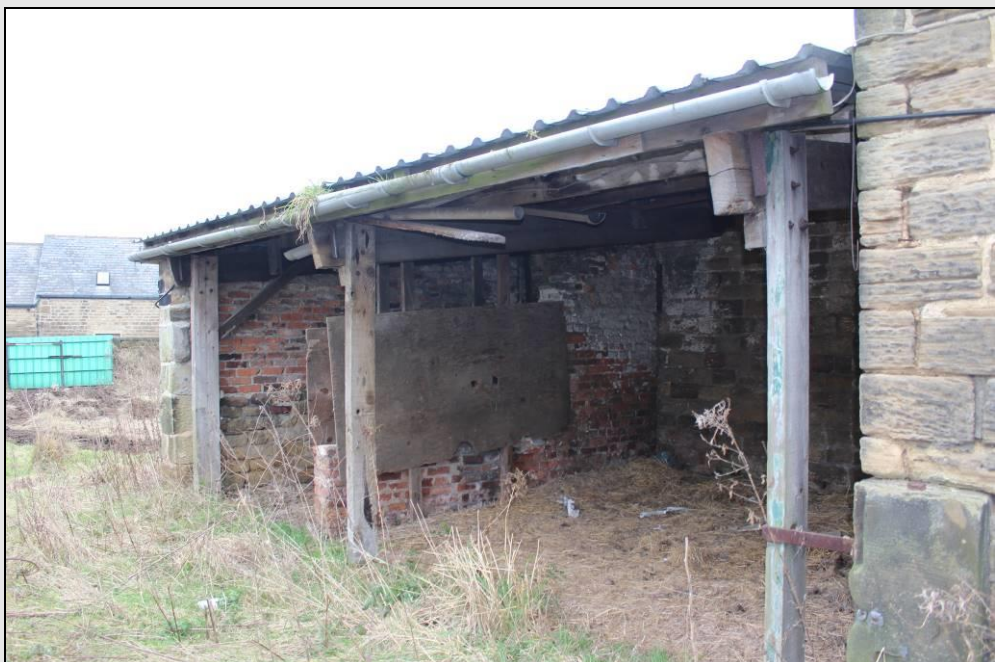
Figure 33. External view of north-west face of Building 3C.
