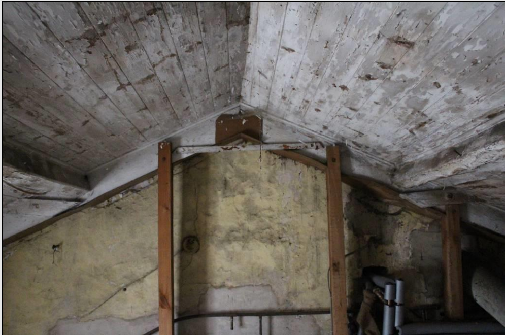
Figure 15. View of loft space inside Building 1B, showing tightly fitted sarking.
