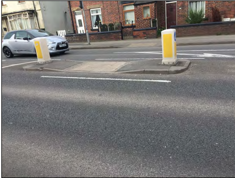
Image 2.5 Pedestrian Refuge Island on A61 Sheffield Road
