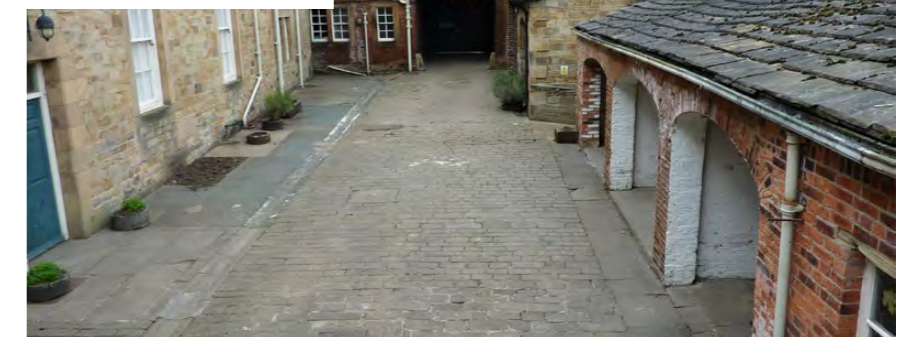
Service wing courtyard
