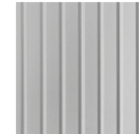
Vertical asbestos cladding
