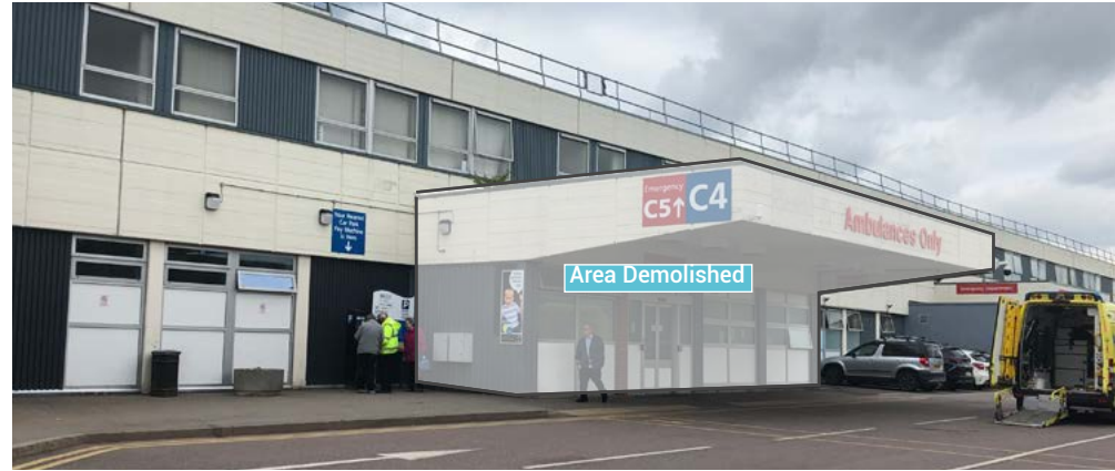
North Facade & Demolition
