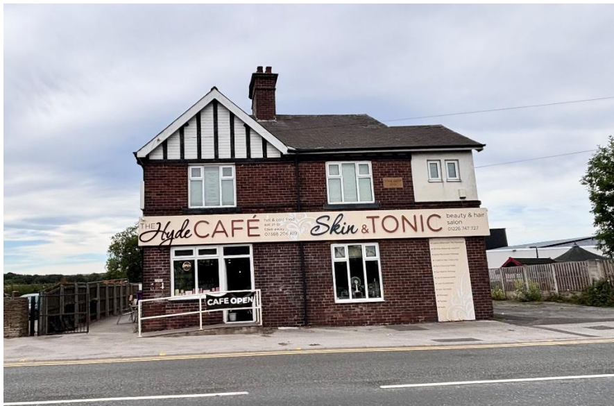
Figure 5 Tankersley Mine Rescue Station from principal east elevation
