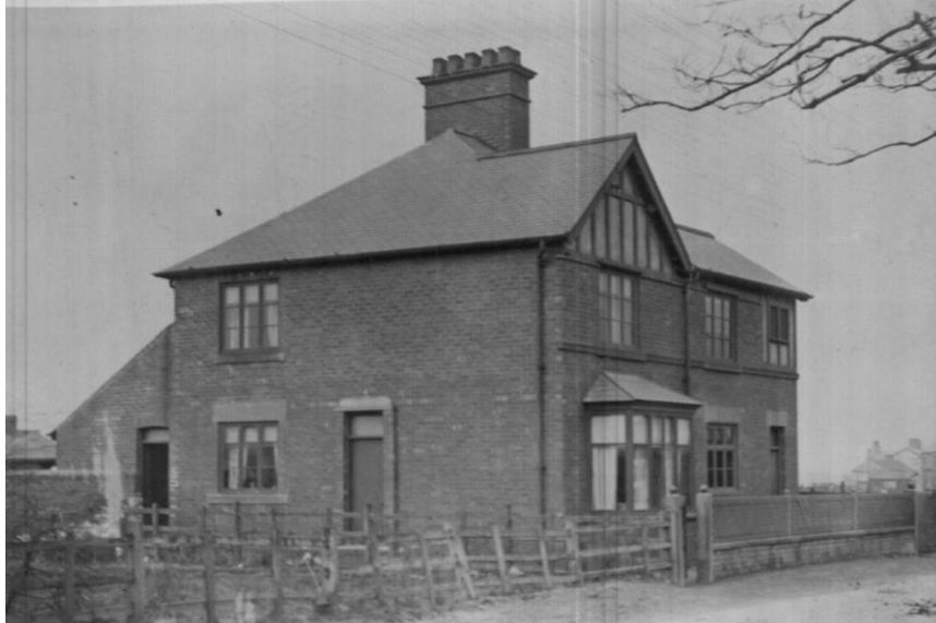
Figure 3 1902 photograph of the station. Image: MRS Training and Rescue.
