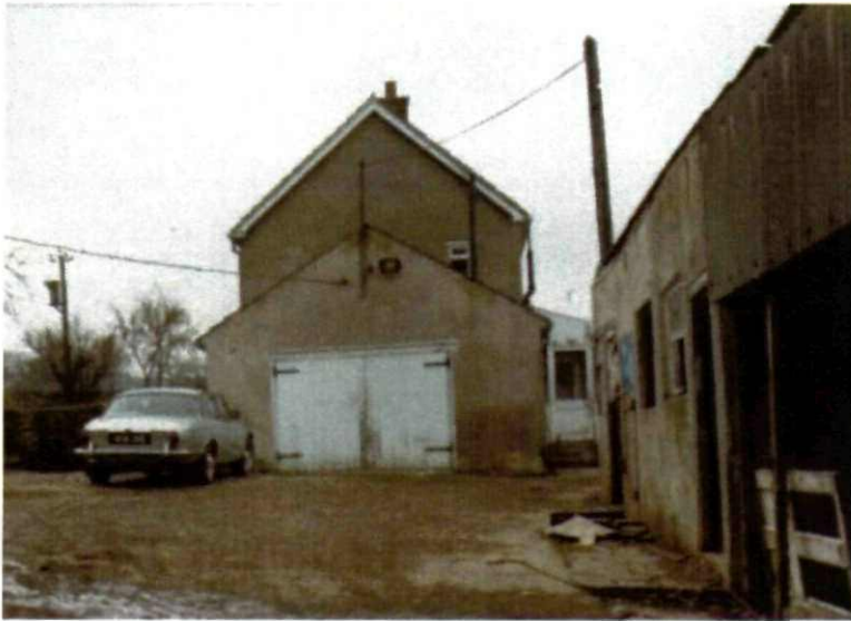
Figure 20 - Photo of North elevation (circa 1980)
