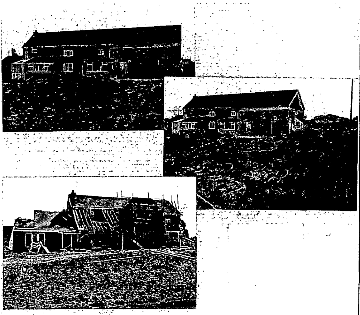
Figure 7 - Front of house (West elevation) in 1980's after demolition of outbuildings, and during construction of extensions
