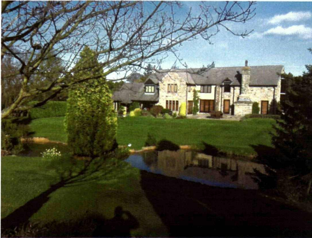
Figure 8 - Front of house (West elevation) as existing (2011)
