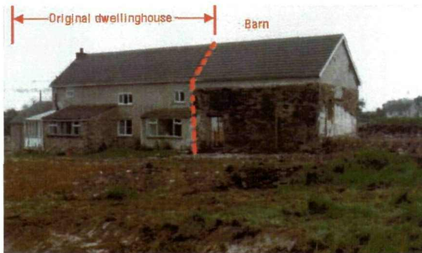
Figure 16 - Annotated photo of West elevation after demolition of cow shed & outbuildings (1980's)
