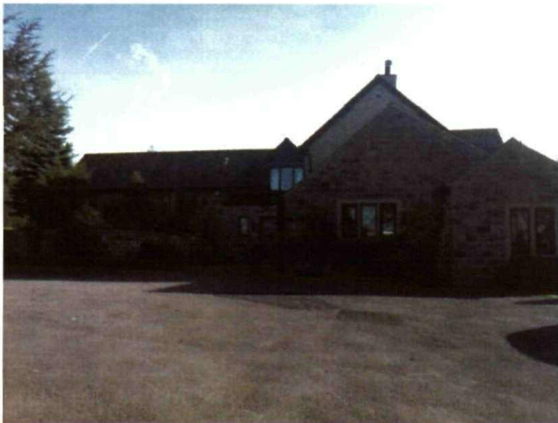
Figure 21 - Photo of North elevation (2011)
