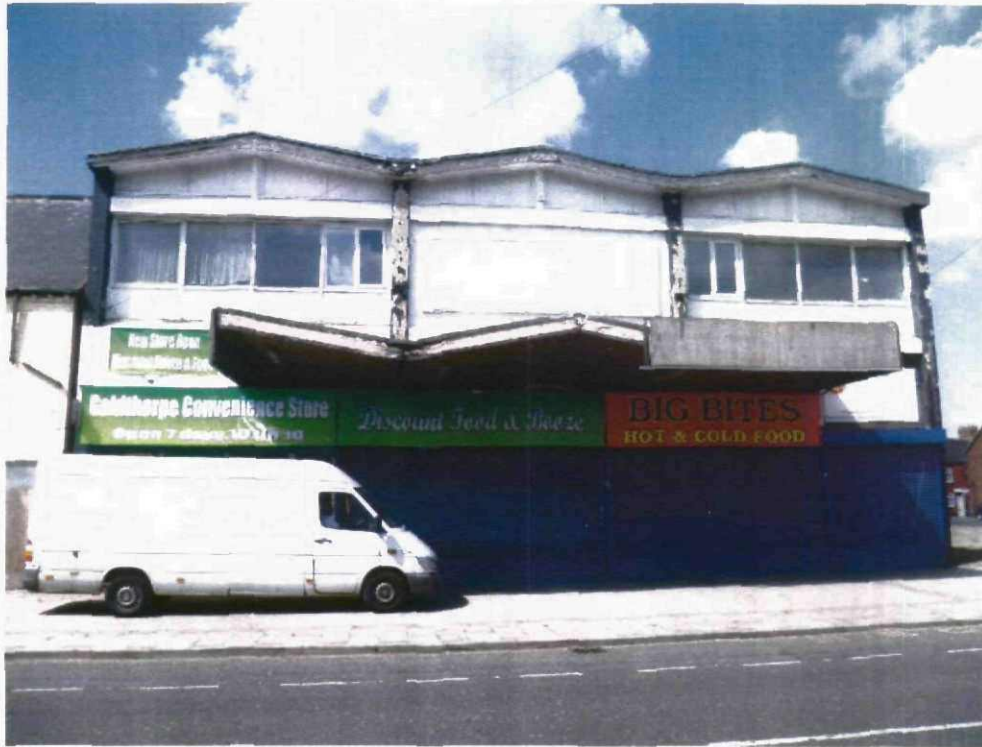
View of existing south elevation to Doncaster Road
