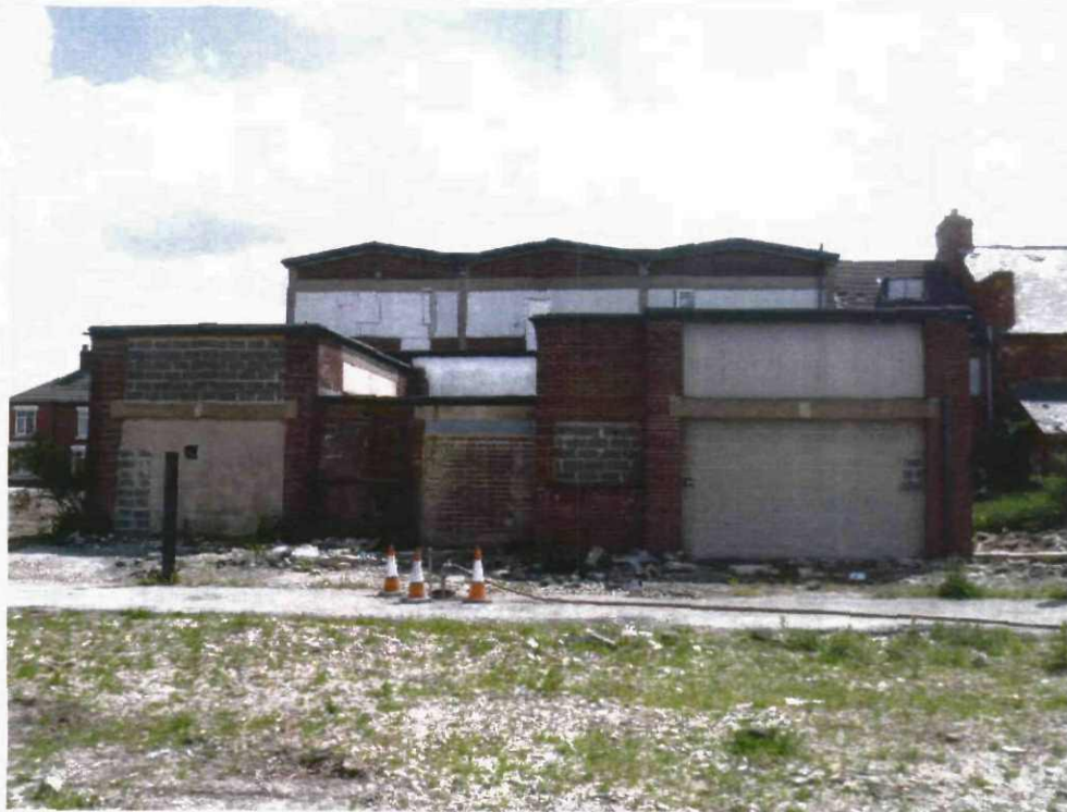
View of existing north elevation
