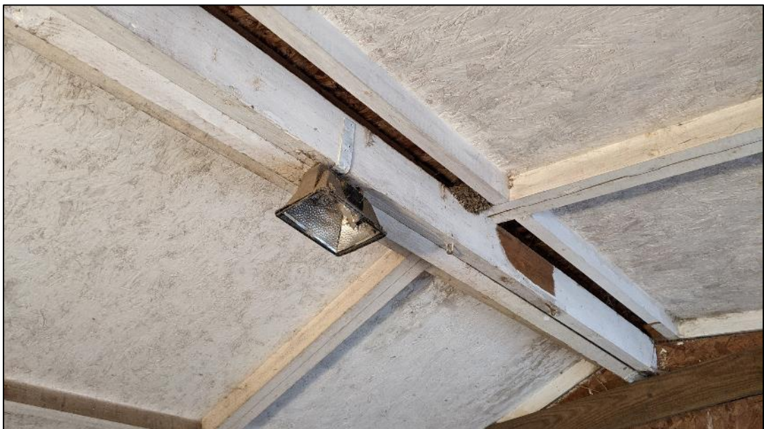
Plate 4. Interior of roof with old swallow nest visible
