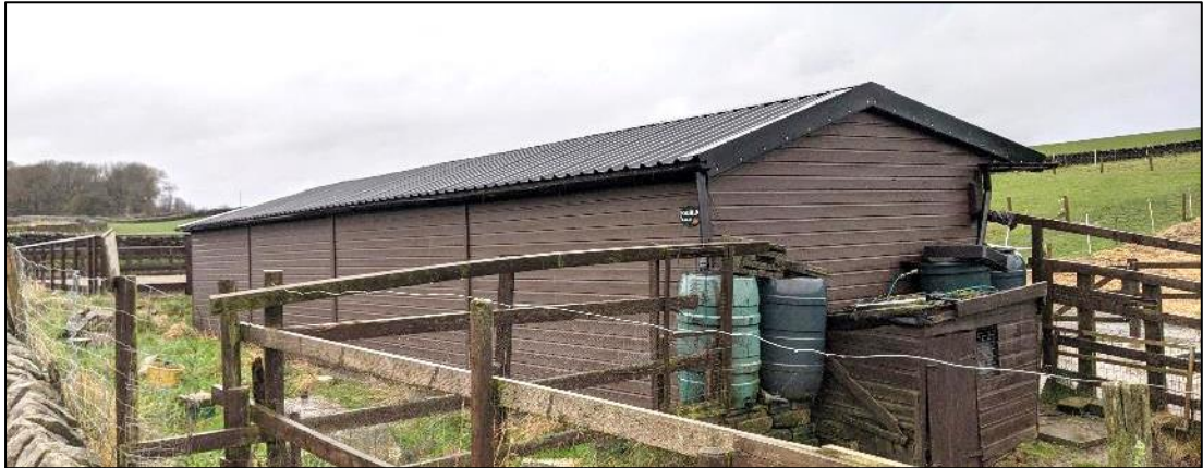
Plate 3. Southeast corner of stables
