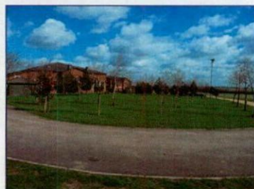
② View facing North East of the rear of the Hotel facilities and existing track between Hotel and 'The Qube'.
