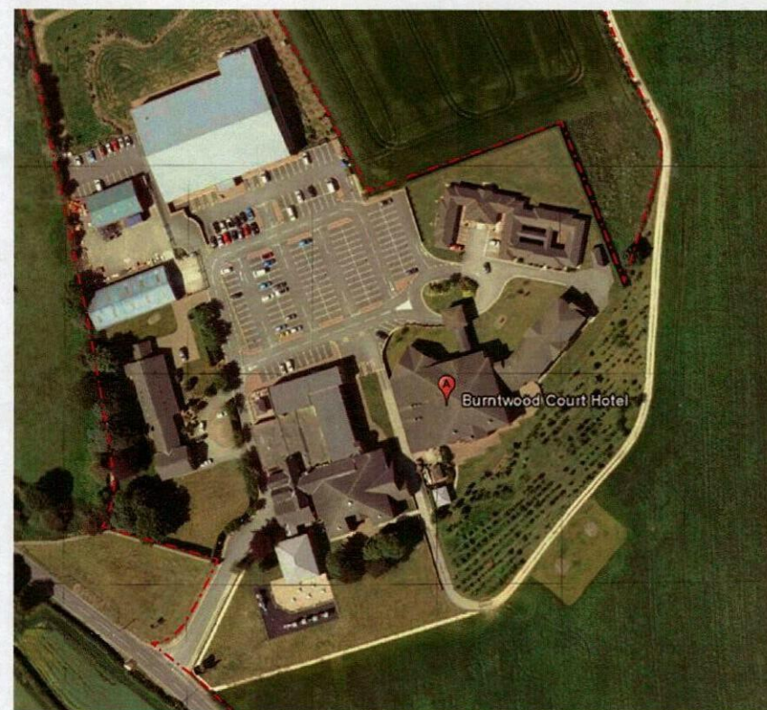
Figure 1: Aerial image showing the Burntwood Court complex and location of ownership boundary.
