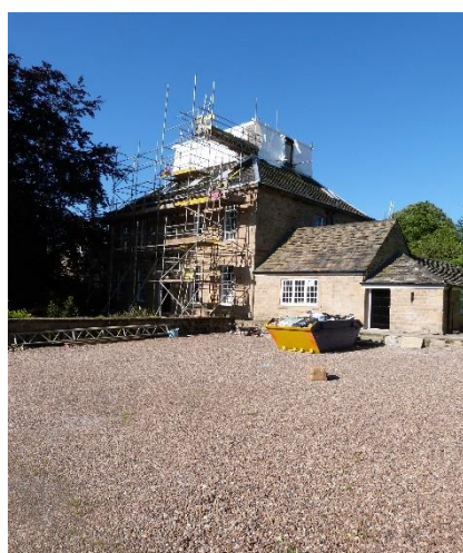
Image 2. East front during repairs.
