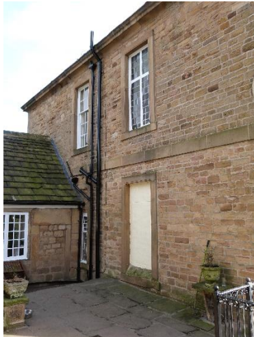
Image 6. Blocked window in courtyard.
