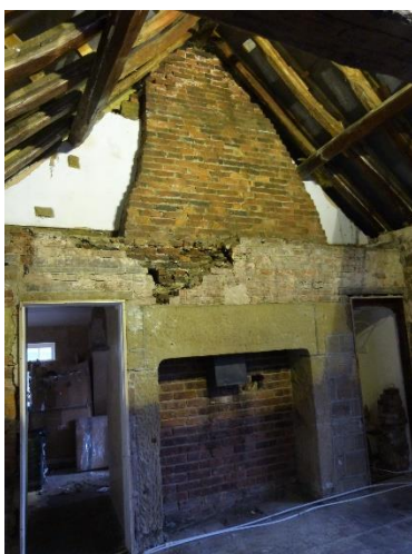
Image 10. Kitchen fireplace phase 1.
