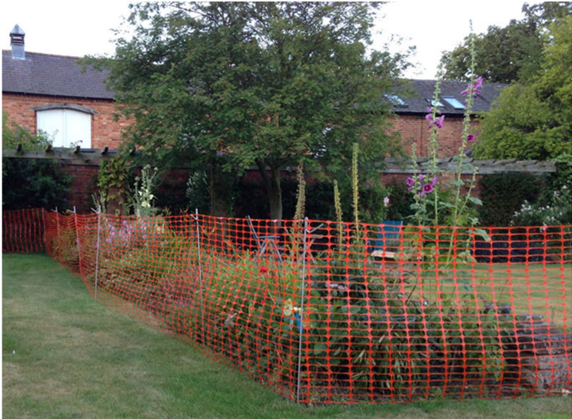
Figure 4: Plastic mesh fencing secured with heavy duty metal stakes
