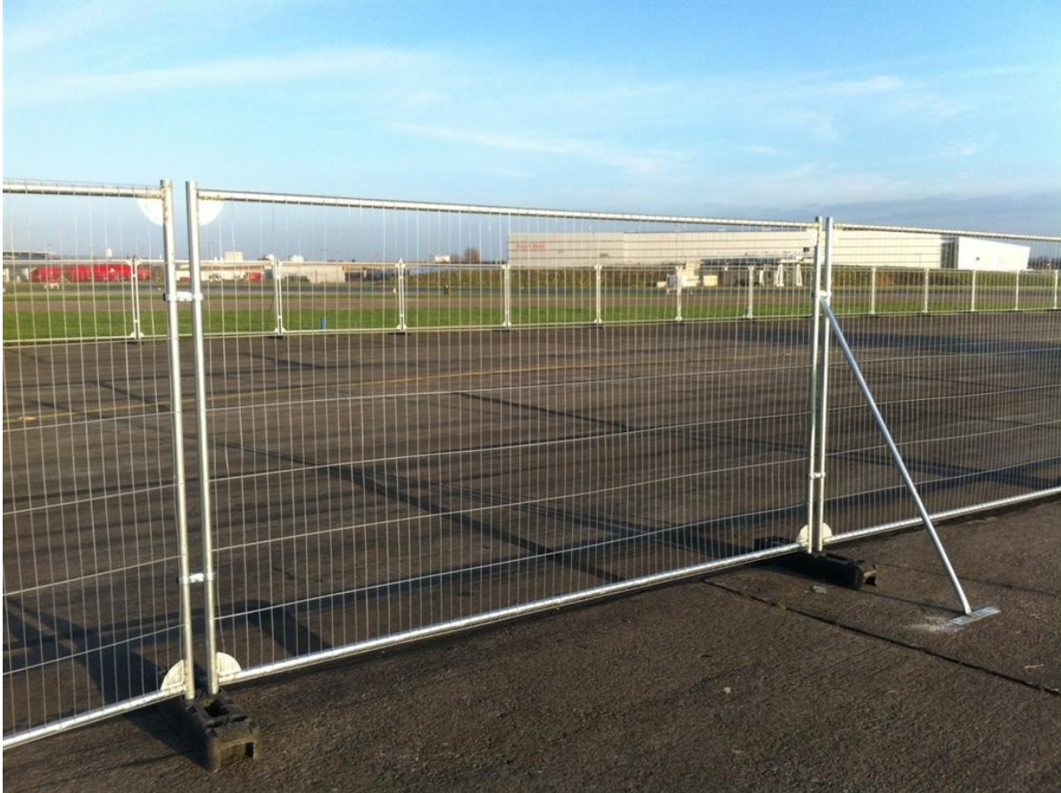
Figure 2: Secured 'Heras' type fencing with stabilizing system and anti-tamper couplers
