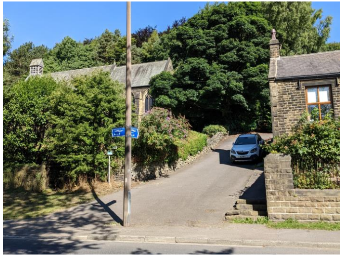
TPT access to left of No.213 Manchester Road
