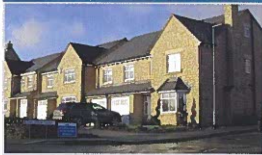
Photo 5 – Existing Finishes on Wellthorne Lane
