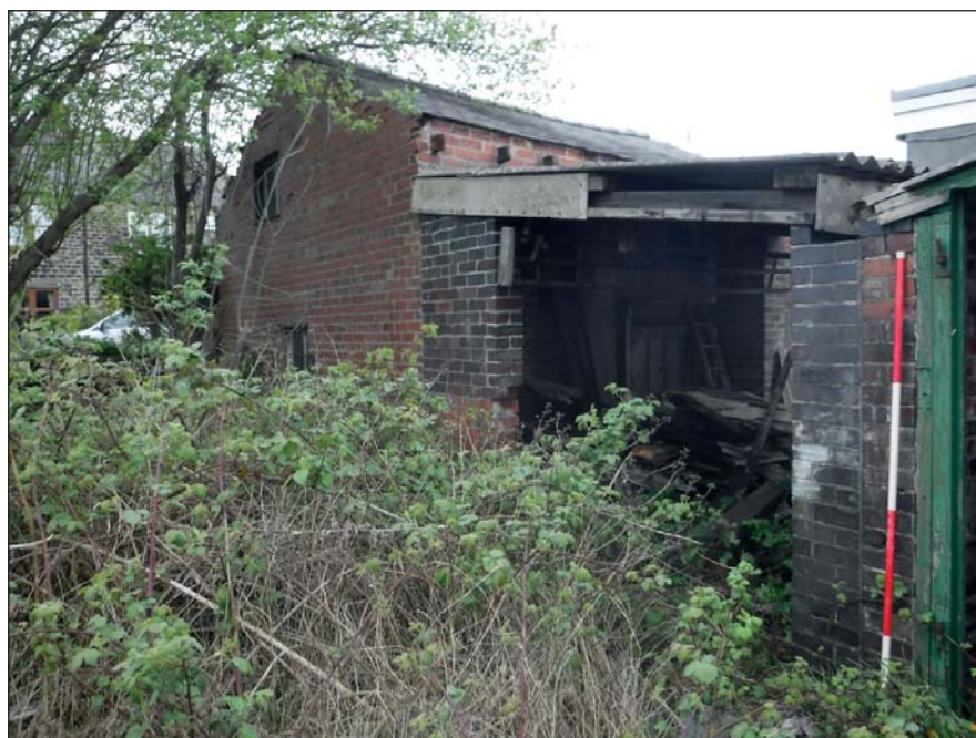
Plate 4. Structures on northern part of site, looking north
