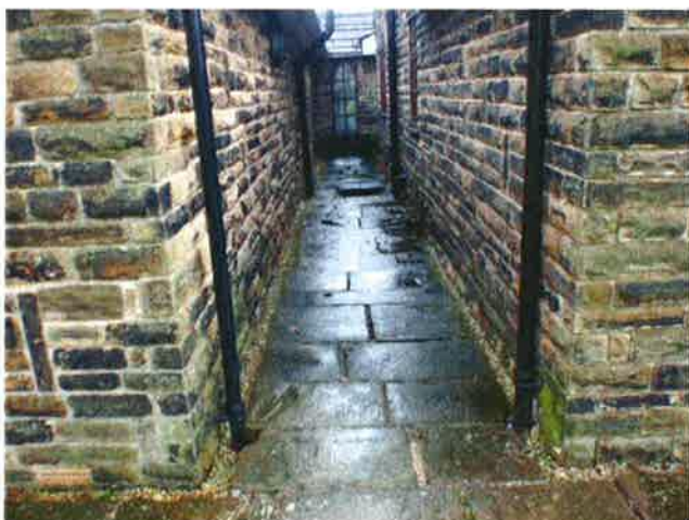
Fig 1.1 – Area Of Surveyed Drainage
