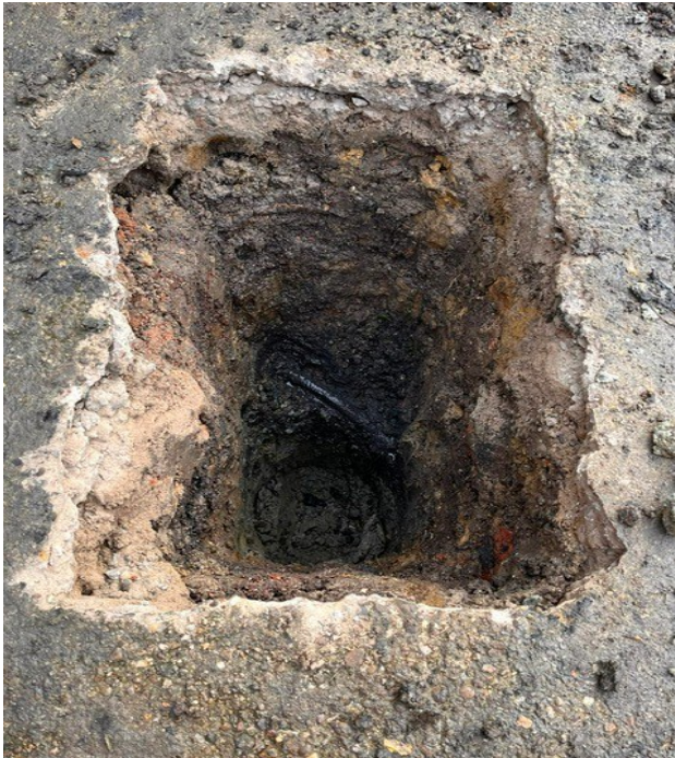
Fig 5 – Pre-drilling Test Pit – Borehole BH1
