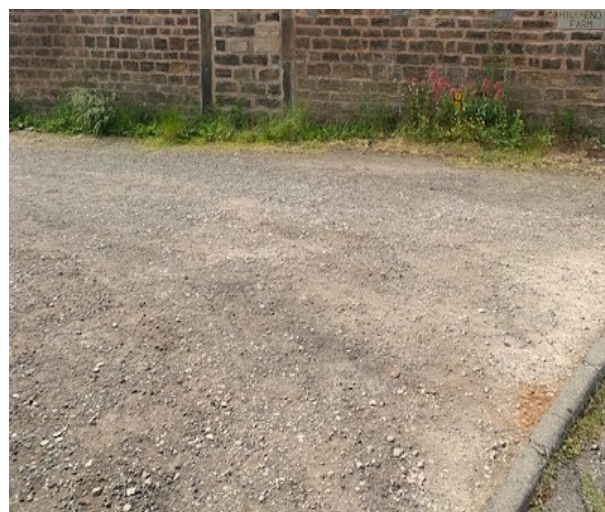
Fig 14 – Front access track and hard-standing
