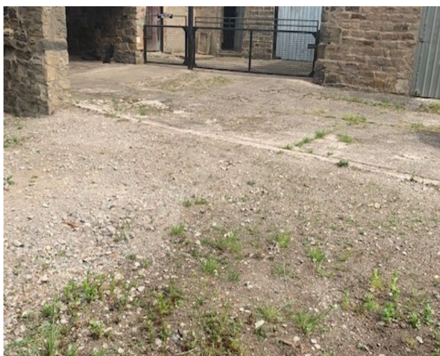
Fig 13 – Rear hard-standing & concreted curtilage
