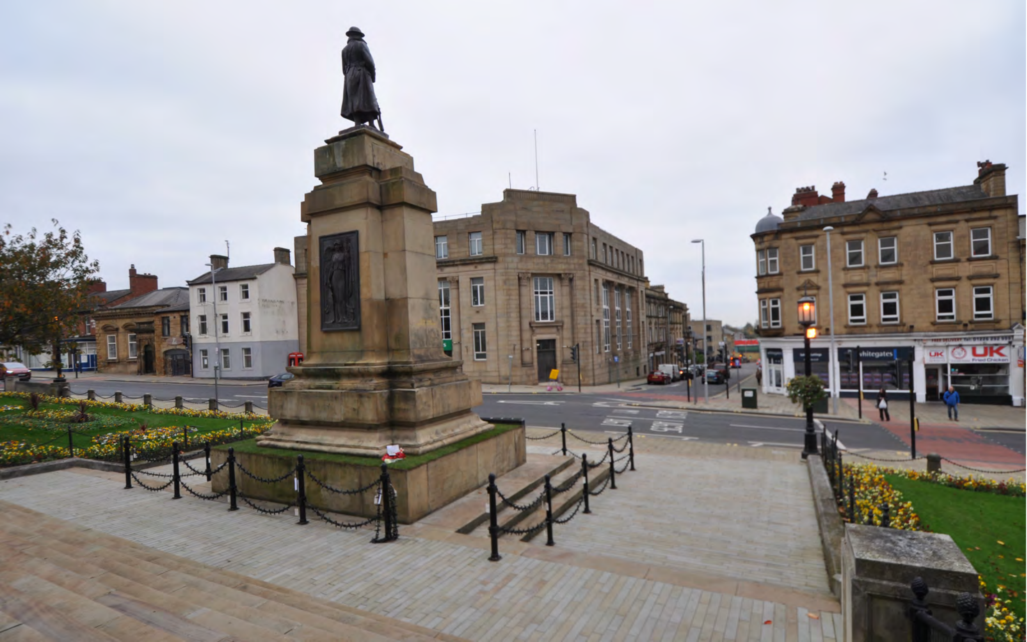
View towards the site from outside the Town Hall with the Grade II* Listed War Memorial in the foreground. There should be no perceivable difference to this view caused by the scheme.
