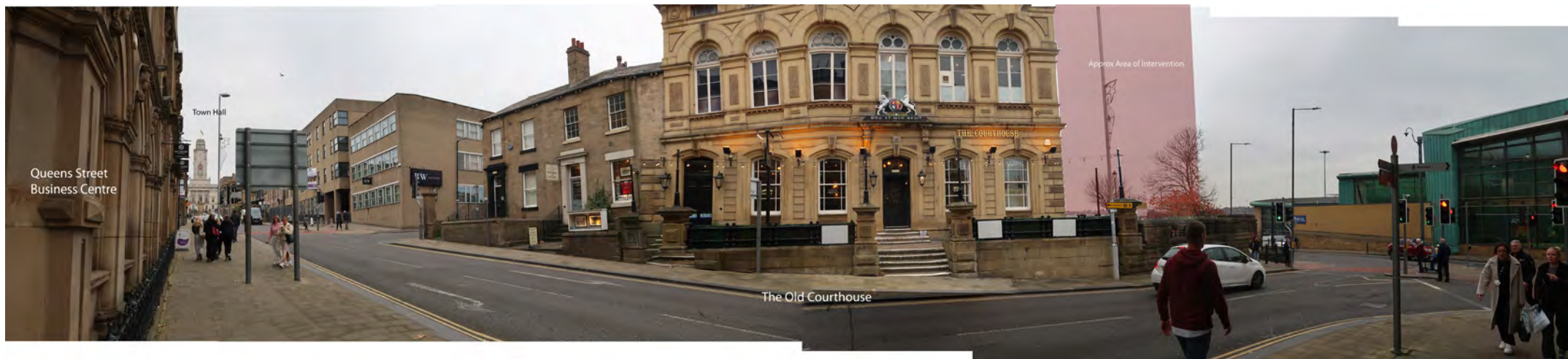
View from Regent Street opposite The Old Courthouse. The site is to the right of the Listed Building and would likely remove attention from the plethora of highway lamp columns and traffic lights to the area's benefit.
