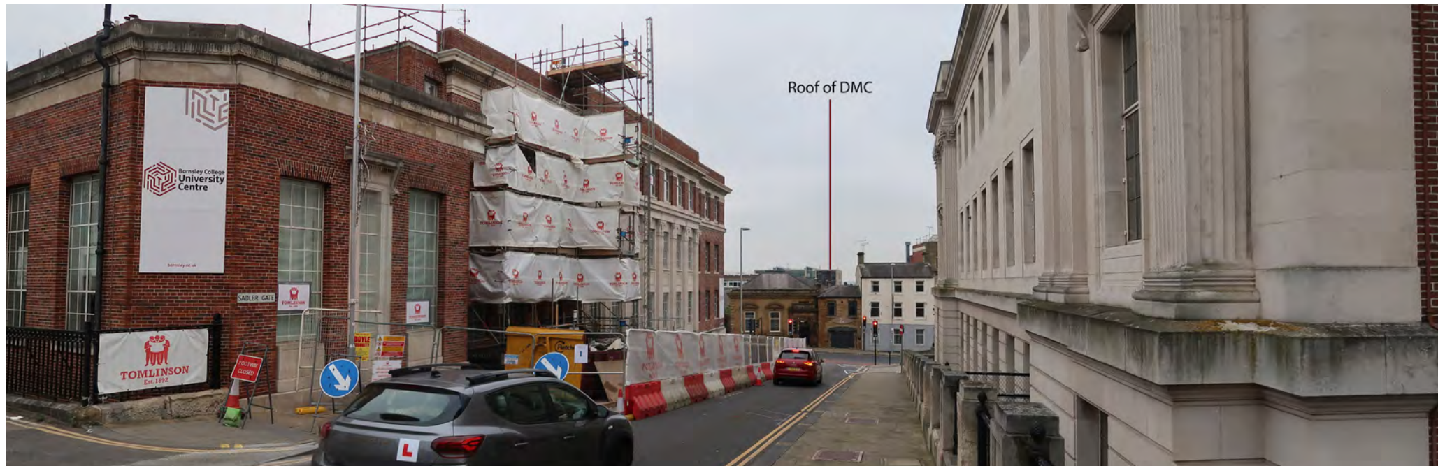
View towards the site the Town hall area looking along Sadler Gate. The roof of the DMC is visible and, although unlikely, there could be the possibility that some of the structures could be visible from here between the gaps in the roofscape. However any such encroachment over the skyline here would be a very minor glimpse and would not affect the significance of the flanking heritage assets seen in this image.
