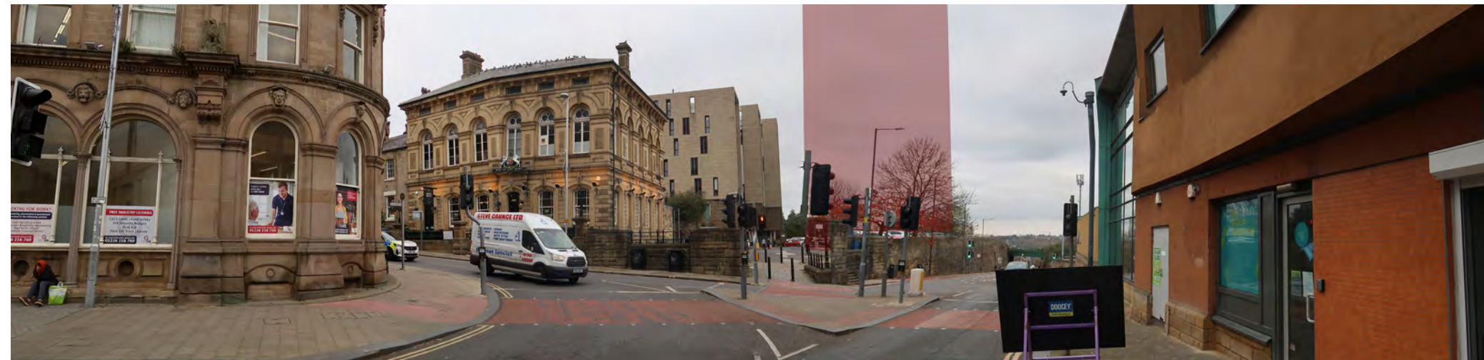
View of the site from near to the junction of Eldon Street and Regent Street with the Old Courthouse and DMC visible. The art works would be visible from here and become something of a landmark. Their contrasting architectural nature and quality would help enhance the townscape here.
