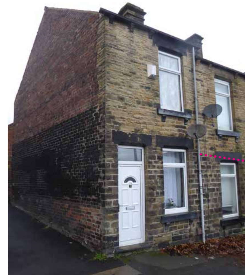
figure a - typical terraced house. Stone facing is graduated above ground floor with smaller format coursing
