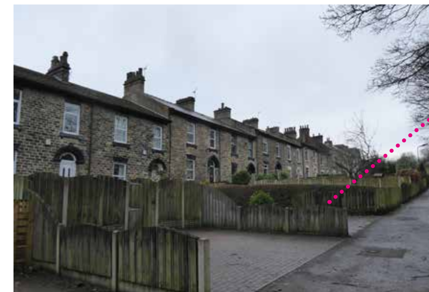
figure b - Properties facing towards Locke Park, have finer details around the front door and roofs are stepped in pairs of houses
