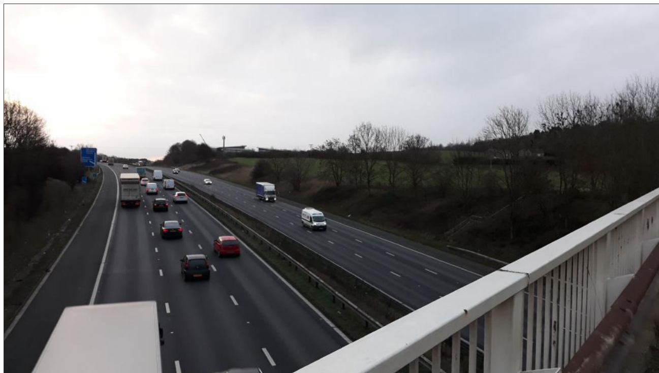
Photograph 9: M1 motorway, looking southeast towards the site.
