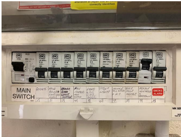
Image 23 Distribution/fuse board
