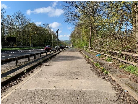
Image 9 View of Layby & concrete filled weighbridge
