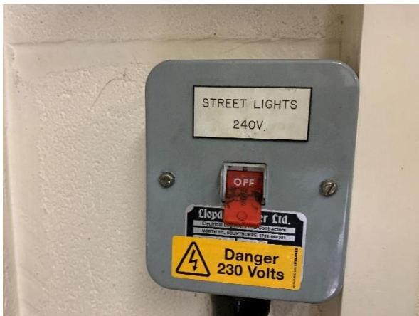
Image 19 External Light Controls
