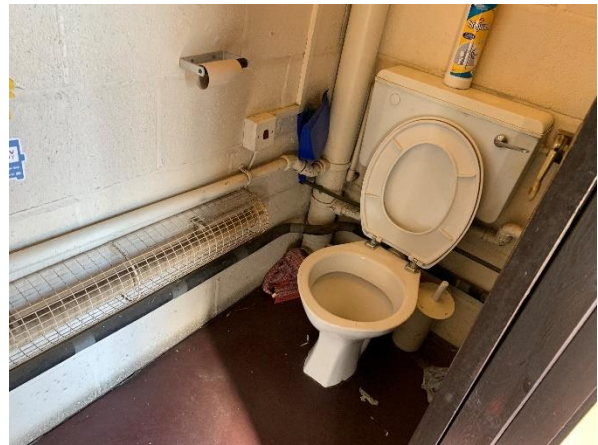
Image 24 Toilet and electric wall heater
