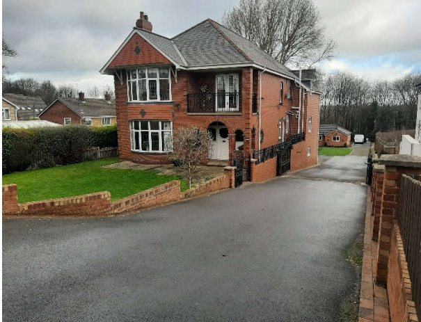
Photo 1: 73 Park Street, as viewed from the highway to the south
