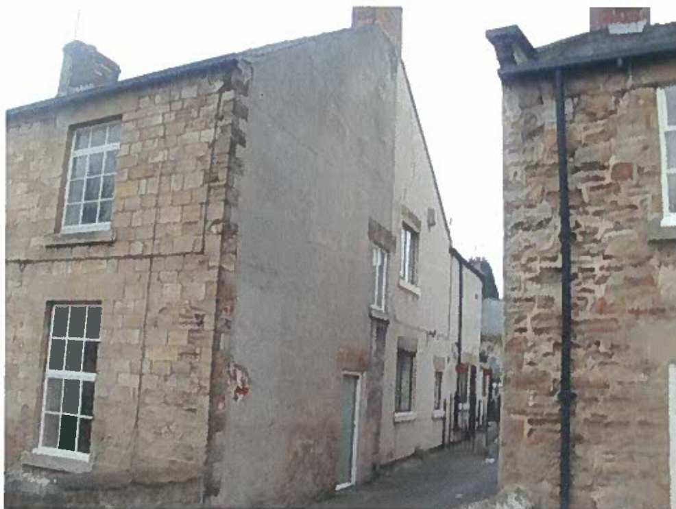
Photo 5- Gable to 102 Wath Road
