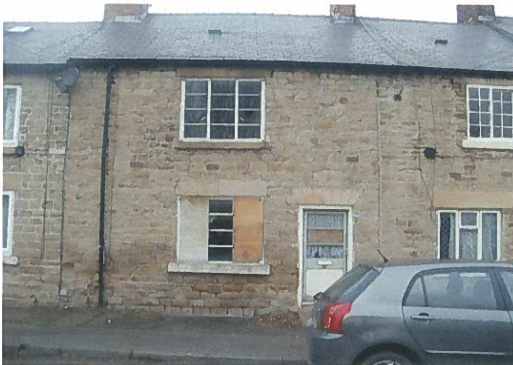
Photo 2 – Front Elevation 98+100 Wath Road
