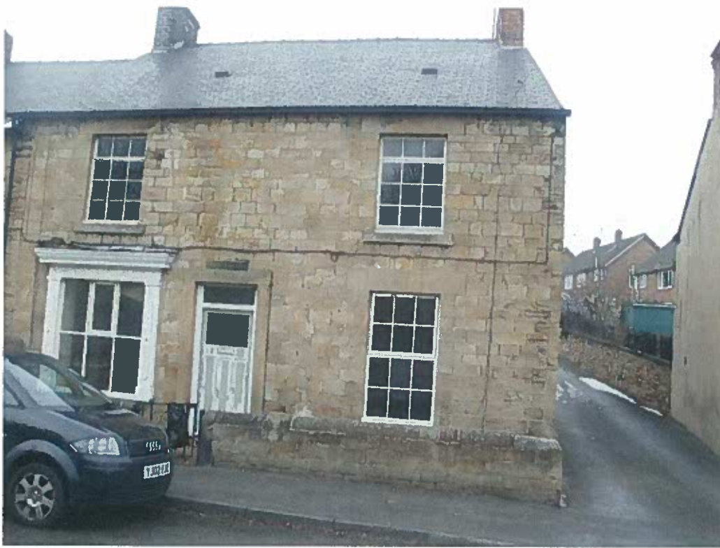
Photo 1 –Front Elevation 102 Wath Road
