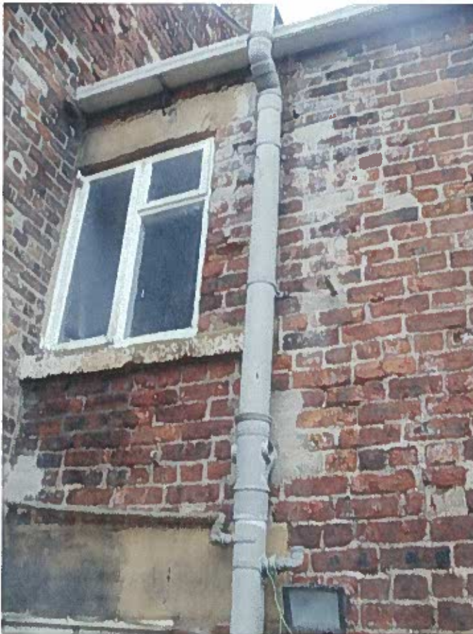
Photo 10- Rear Elevation 100 Wath Road First Floor
