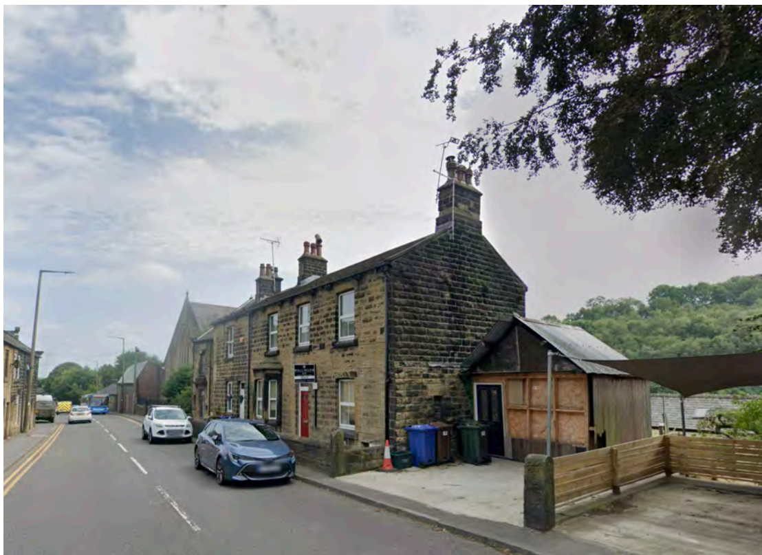
Building Frontage Manchester Road
