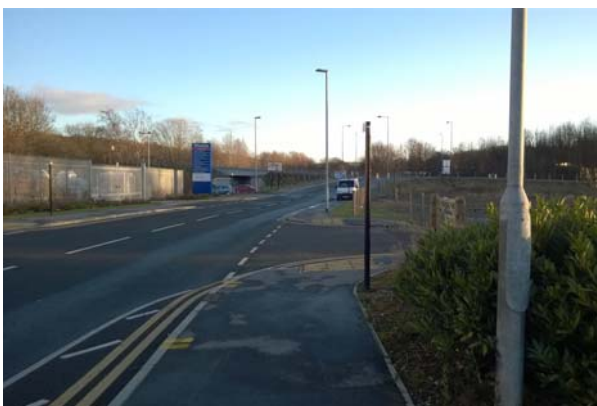
Site Access Road towards the existing roundabout
