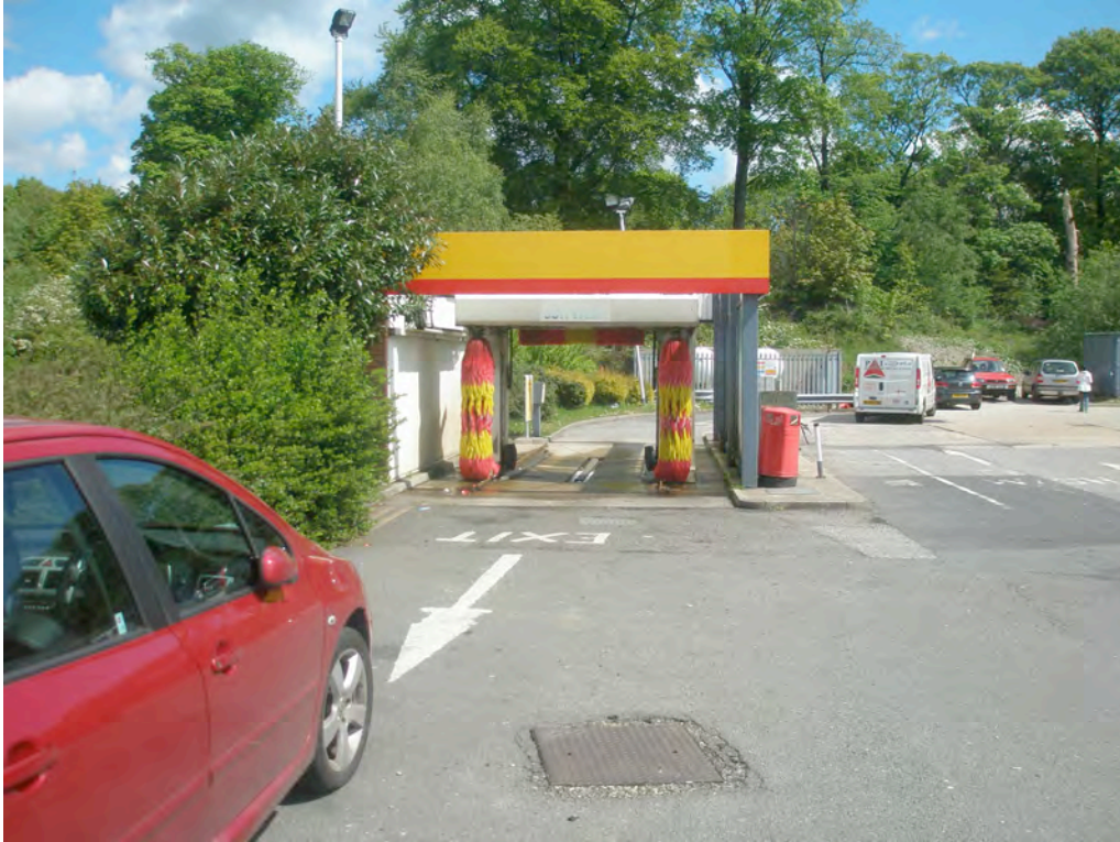
Existing Car wash to be removed
