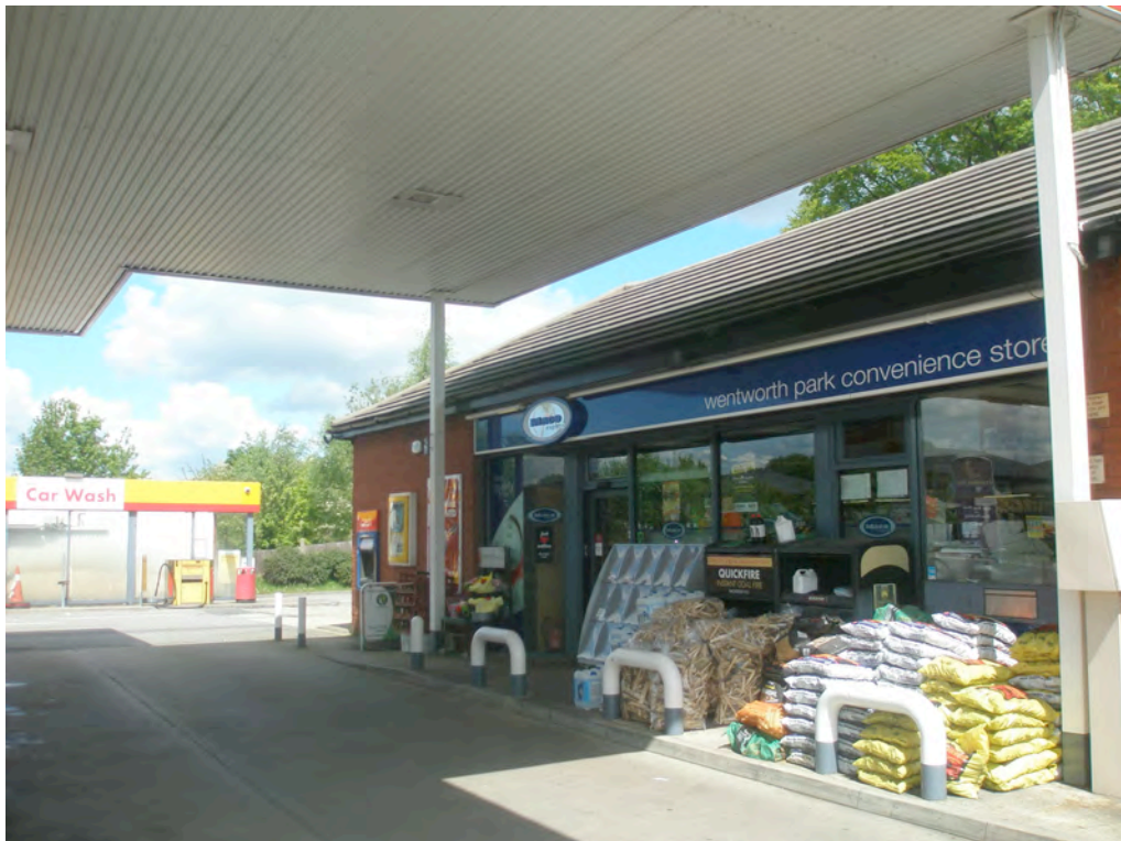
Existing sales building in need of upgrading and refurbishment
