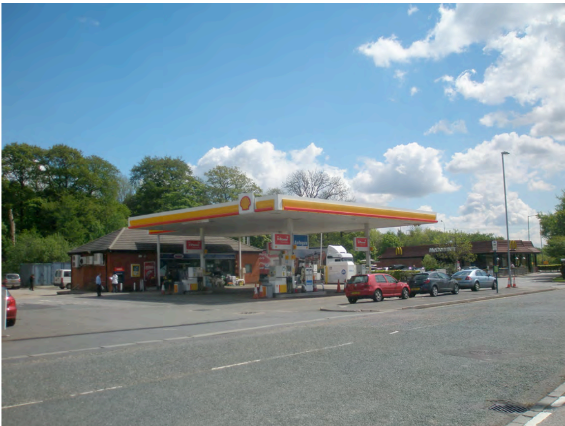
Wentworth Service Station
