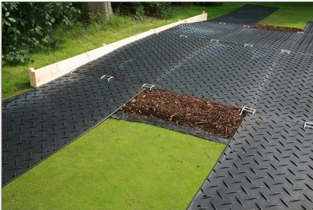
Figure 3. An example of suitable temporary ground protection spanning over a root protection area.
