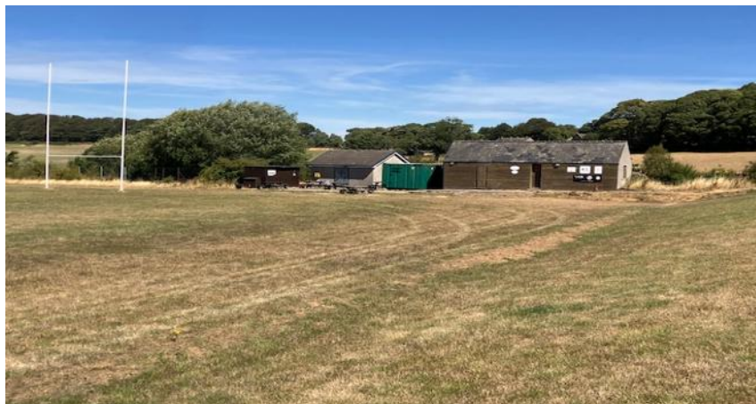
Wortley RUFC Changing Rooms, Shower container and Toilets. Looking north.
