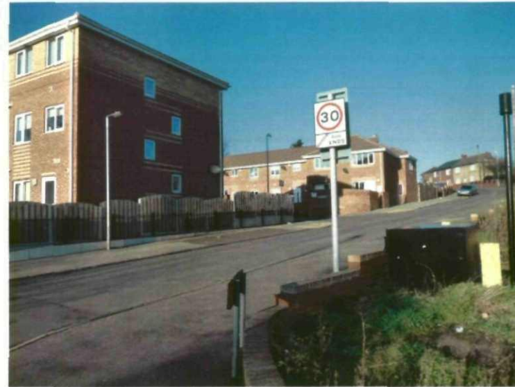
Photo 03: Adjacent properties on Tudor Street
