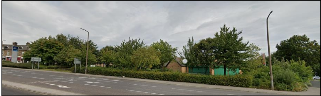
The site viewed from the South West across the main Doncaster Road A365 dual carriageway
