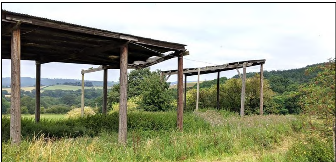
Plate A6.16. Building 7 is located on right of image with B8 on left
