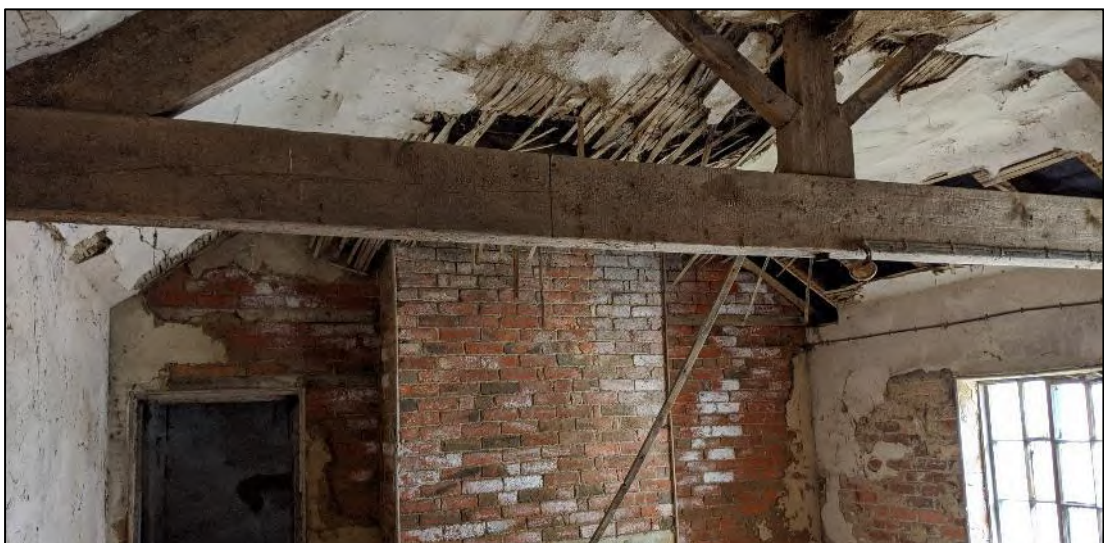
Plate A6.3. Interior of B1, in southern section of first floor
