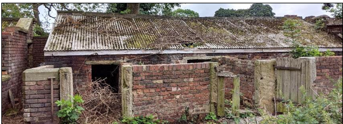
Plate A6.13. Northwest elevation of B5, with B4 on far left of image
