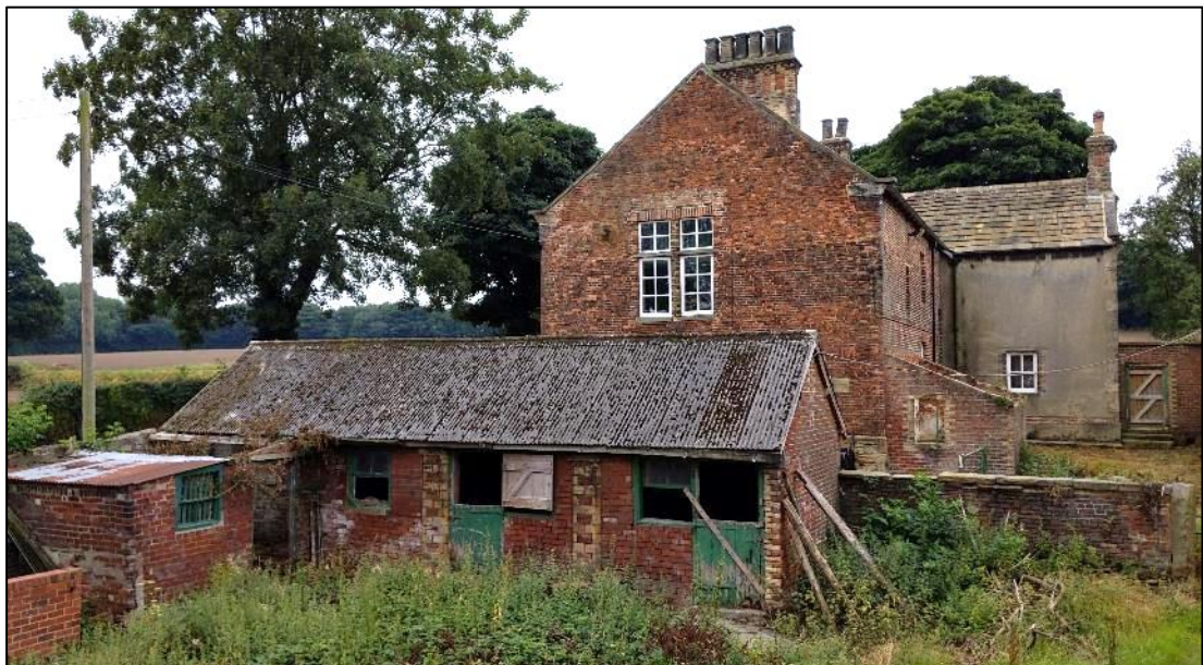
Plate A6.14. Northeast elevation of B6 in foreground with the farmhouse (B11) in background
