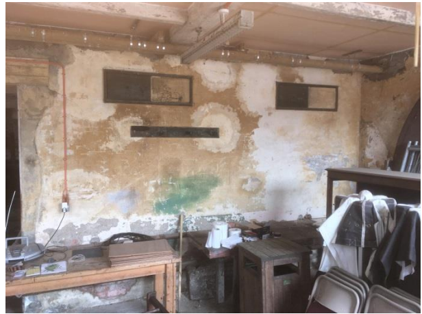
MAIN GARAGE ROOM 2 – RECESS AT REAR TO FORM SERVERY TO CAFÉ. STONE FLAG FLOORS TO BE RELAID, TO OVERCOME TRIP HAZARDS.
