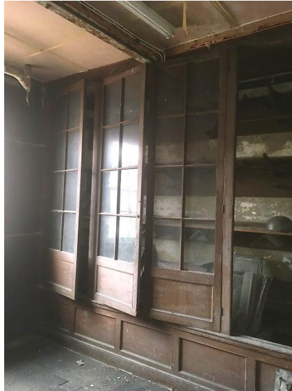
TACK ROOM 4 – PANNELLING, CABINETS AND FITTINGS TO BE RETAINED AND REPAIRED. QUARRY TILED FLOOR TO BE CLEANED AND RETAINED.
