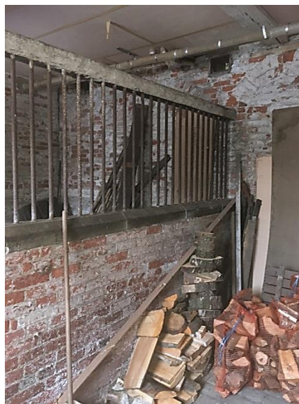
RIGHT HAND STABLE ROOM 1 – STABLE DIVISIONS TO BE RETAINED, STONE FLAG FLOOR TO BE RELAI, TO OVERCOME TRIP HAZARDS.
