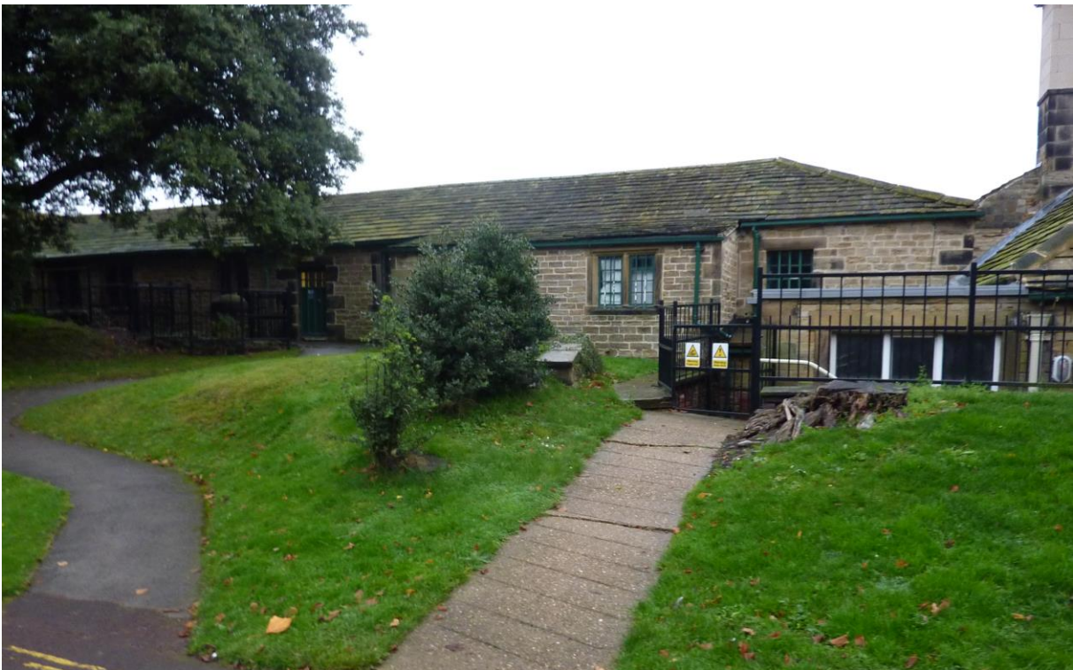
SPENCER WING (UPPER FLOOR OF STABLE BLOCK) VIEWED FROM CANNON HALL FORECOURT
