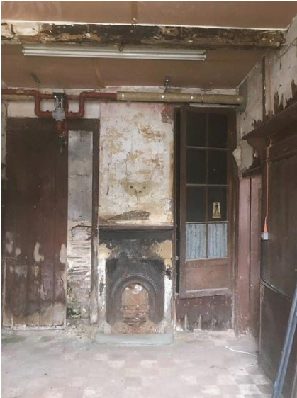
TACK ROOM 4 – PANNELLING, CABINETS AND FITTINGS TO BE RETAINED AND REPAIRED. QUARRY TILED FLOOR TO BE CLEANED AND RETAINED.
