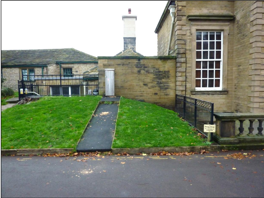
EXISTING LOCATION OF PROPOSED LIFT SHAFT
