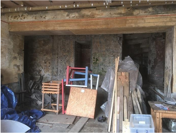
MAIN GARAGE ROOM 2 – RECESS AT REAR TO FORM SERVERY TO CAFÉ. STONE FLAG FLOORS TO BE RELAID, TO OVERCOME TRIP HAZARDS.
