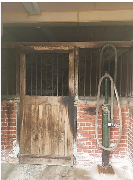
RIGHT HAND STABLE ROOM 1 – STABLE DIVISIONS TO BE RETAINED, STONE FLAG FLOOR TO BE RELAI, TO OVERCOME TRIP HAZARDS.
