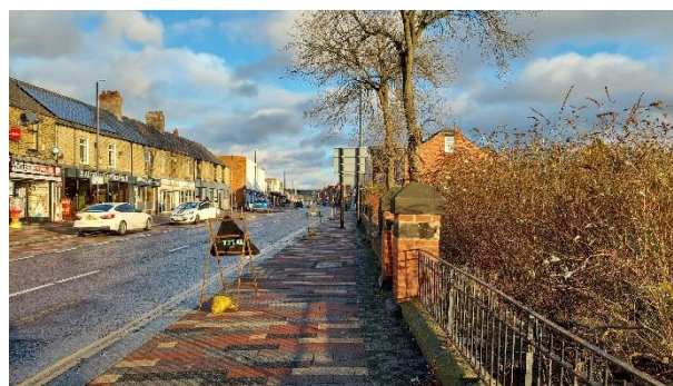
Photograph 10: Photograph taken outside of red line boundary on Doncaster Road but illustrates dense buddleia scrub in the northern section of the site.
