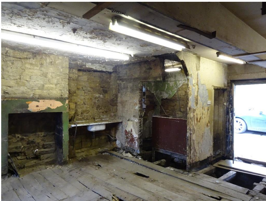
Photograph 4: Inside first floor, showing area where floor is missing under attic entrance
