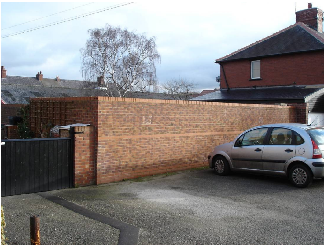
6. Boundary wall between Nos 7 and 9 Park Hill Road looking east.
