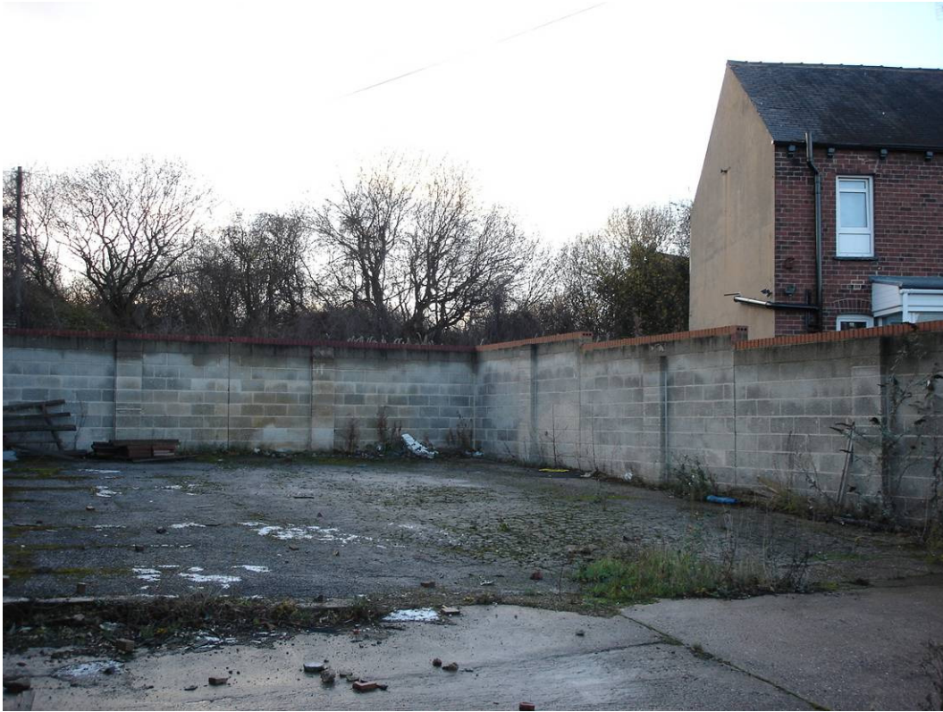
8. Internal view of boundary wall adjacent No 7 Park Hill Road.
