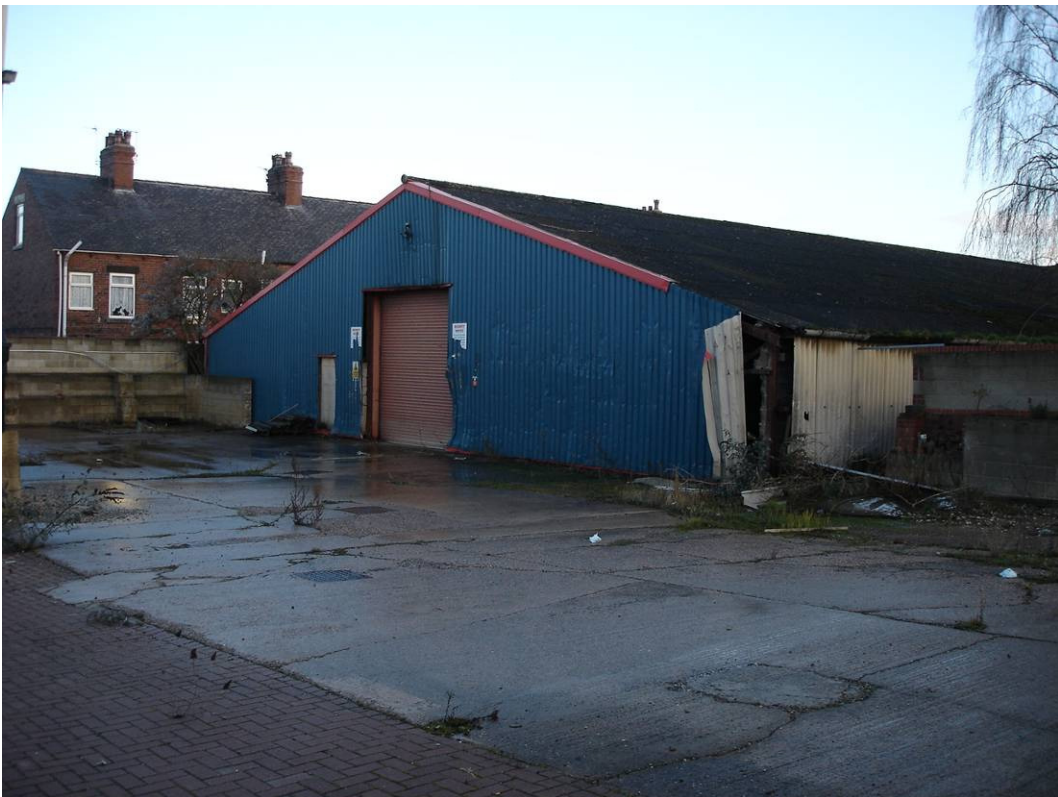
13. Building B – North west elevation with roller shutter.
