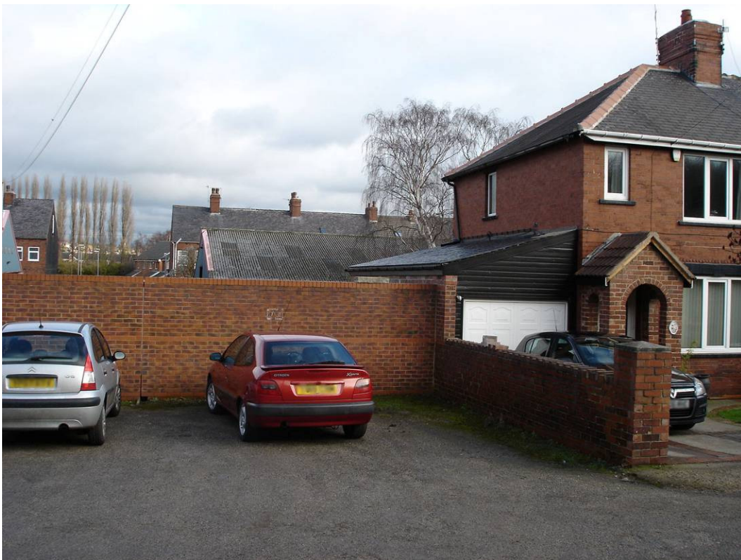
7. Boundary wall adjacent No 9 Park Hill Road looking east.
