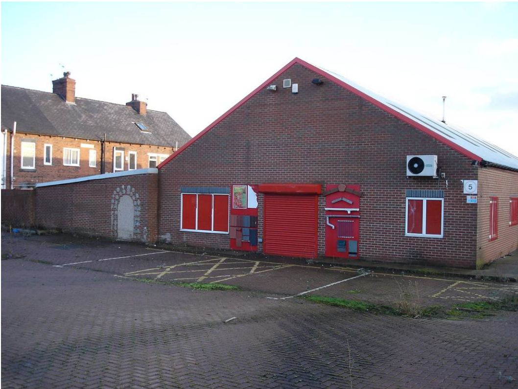
12. Building A – North west elevation.
