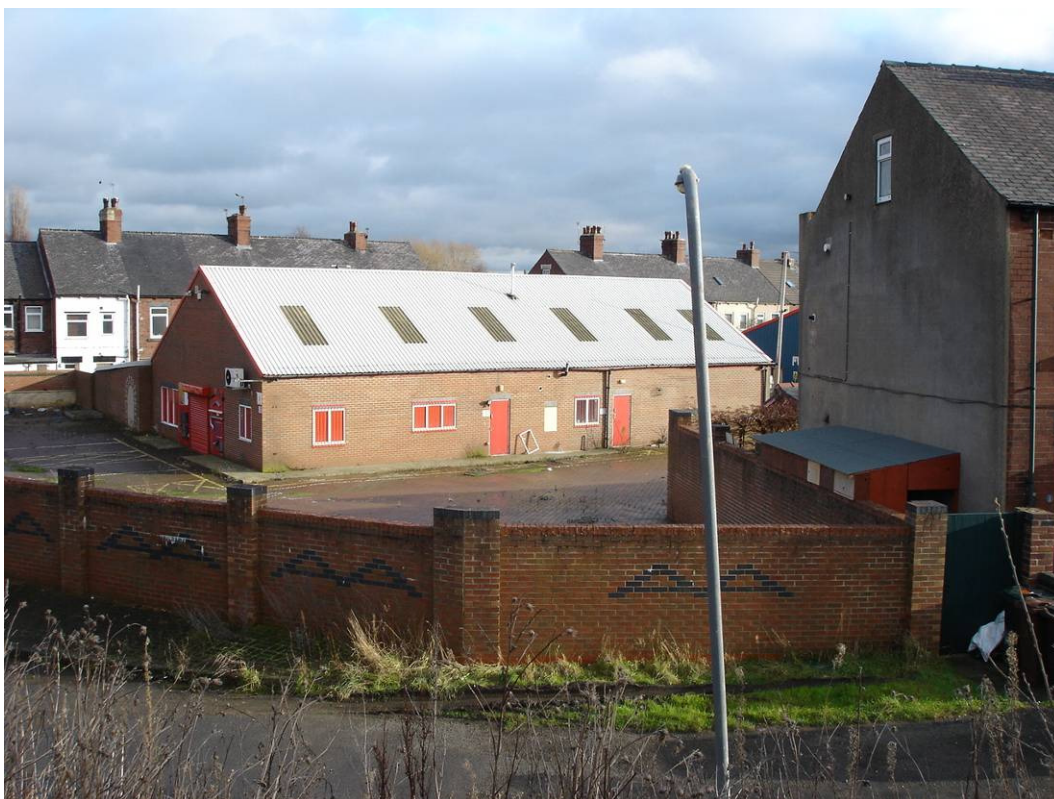
5. Boundary wall and frontage up to boundary with No 1 Park Hill Road.
