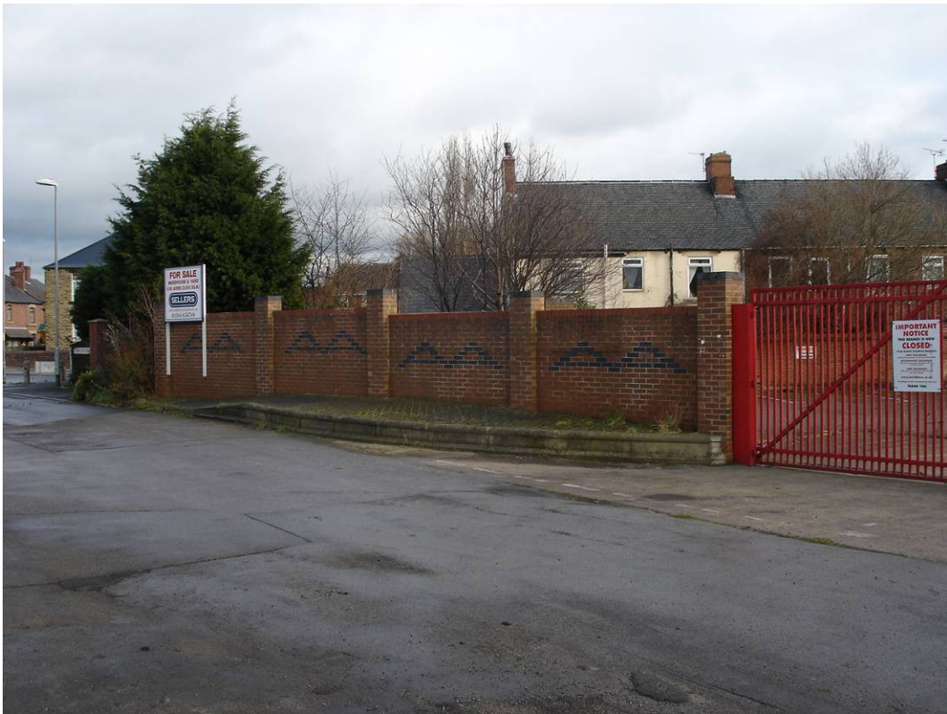
3. Boundary wall and access from Park Hill Road looking north.
