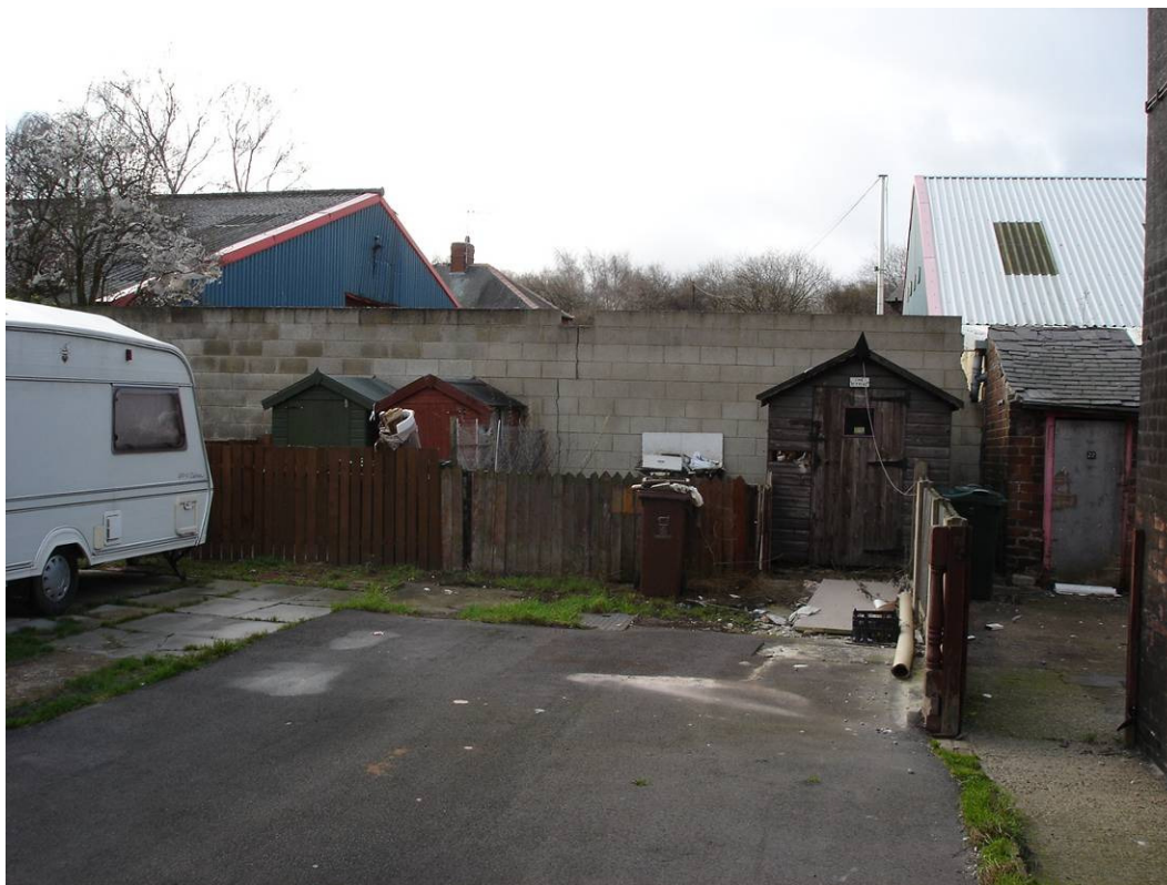
10. External view of boundary wall between Nos 22 and 24 Edward Street looking south west.
