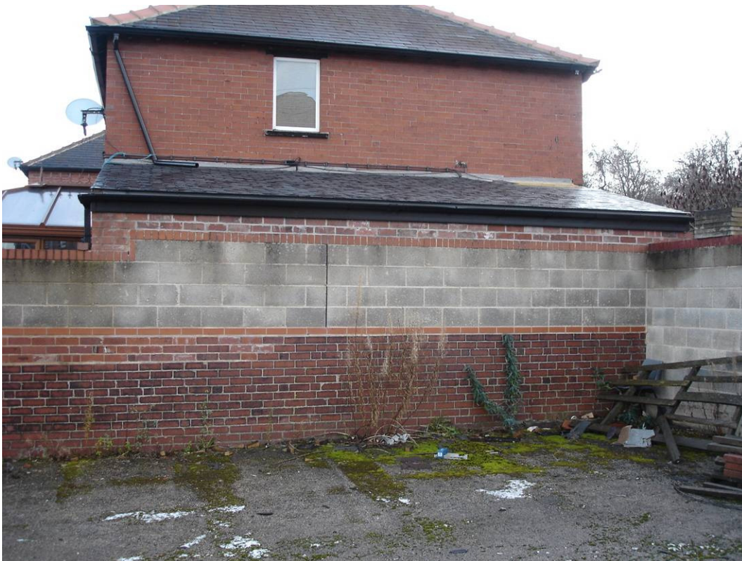
9. Internal view of boundary wall adjacent No 9 Park Hill Road.
