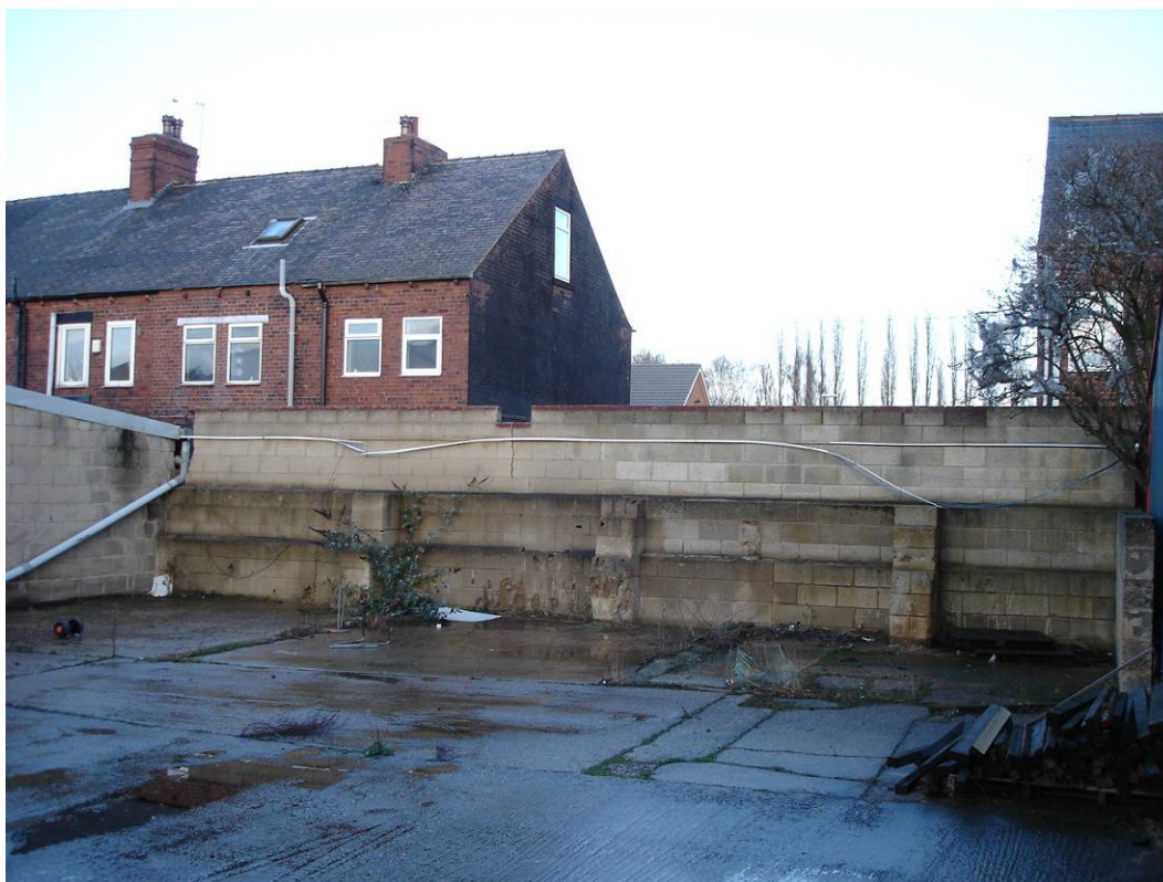
11. Internal view of boundary wall looking towards the rear of No 22 Edward Street.
