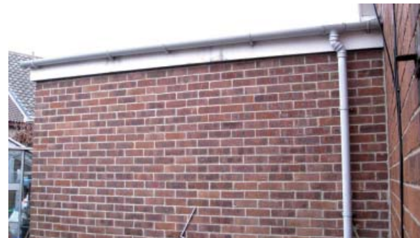
Photo 4 shows existing side extension where new hip roof is proposed
