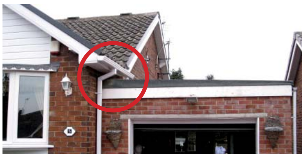
Photo 3 shows conflict area of roof with regards existing eaves
