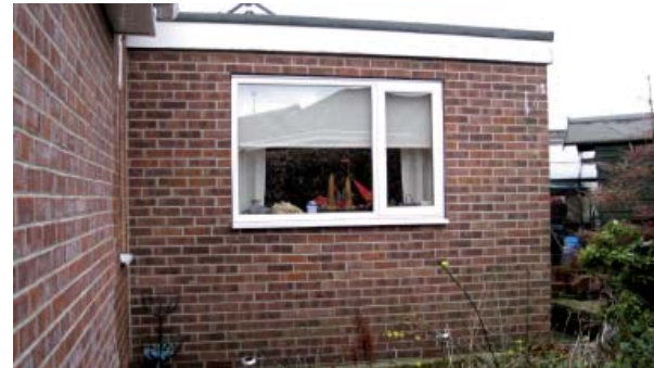
Photo 2 shows existing side extension where new hip roof is proposed
