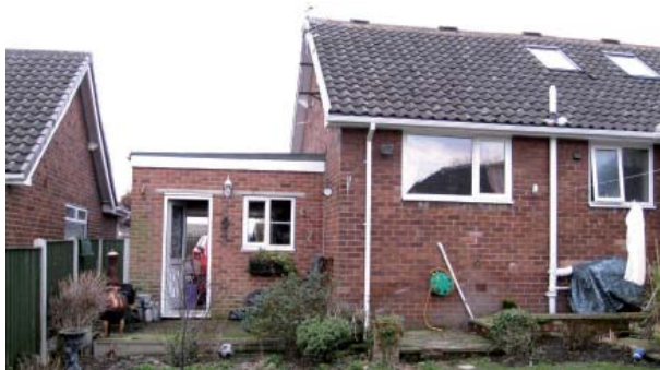
Photo 1 shows rear of existing garage where new utility room is proposed
