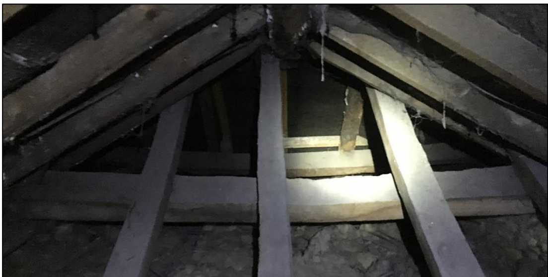
Plate 8. Roof void of dwelling
