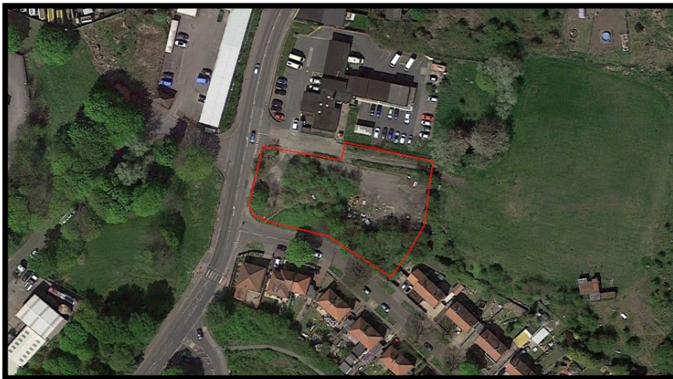
Figure 2: Aerial Image of site (Google Earth)
