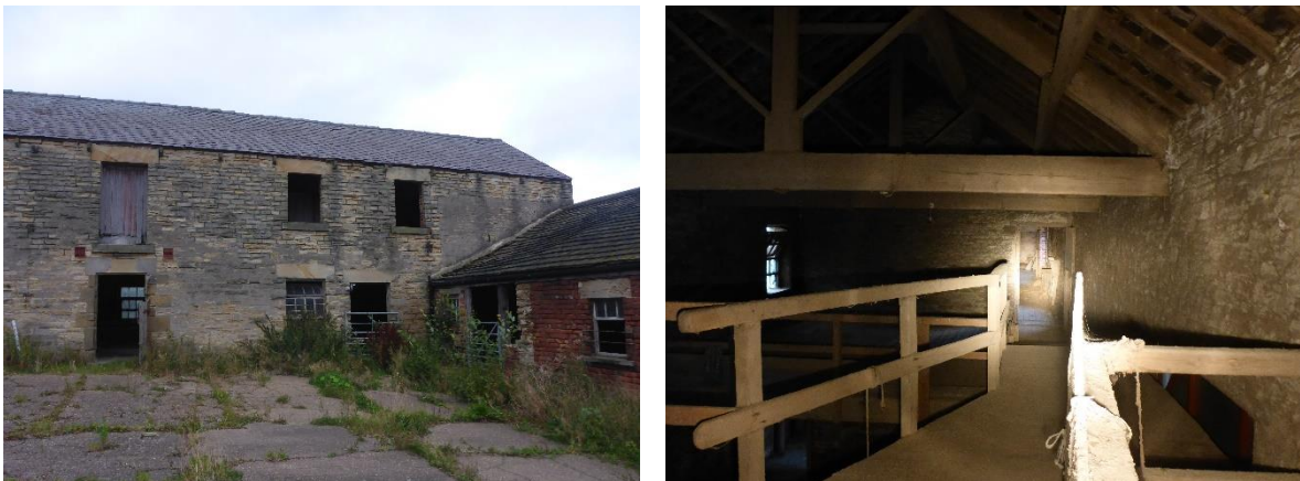
Figure 12 Showing exterior and interior (where safe to access) of Building 6.
