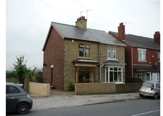
(West of site) Photograph of Victorian/Edwardian Brick and Art.Stone Clad Properties facing Wath Road.
