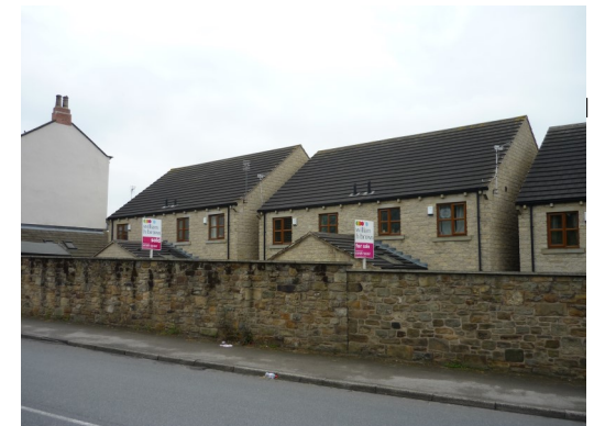
Above (East of site) Photograph shows the rear elevations to recently constructed semi detached dwellings as seen from Wath Road. These properties are constructed of Art.stone.
