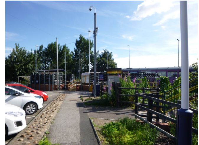
Photo above : Bolton upon Dearne Railway Station.
