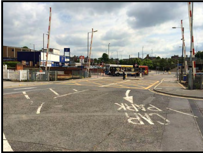
Photograph 2 – Existing Kendray Street level crossing
