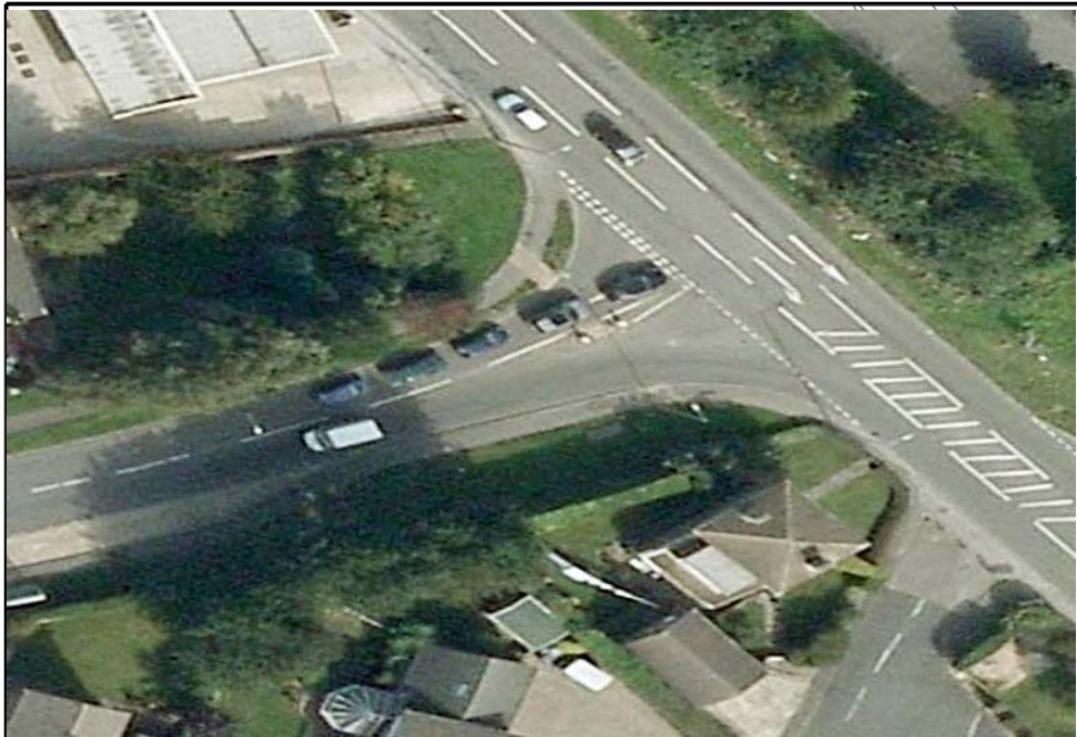
NORTH SOUTH AERIAL VIEW
