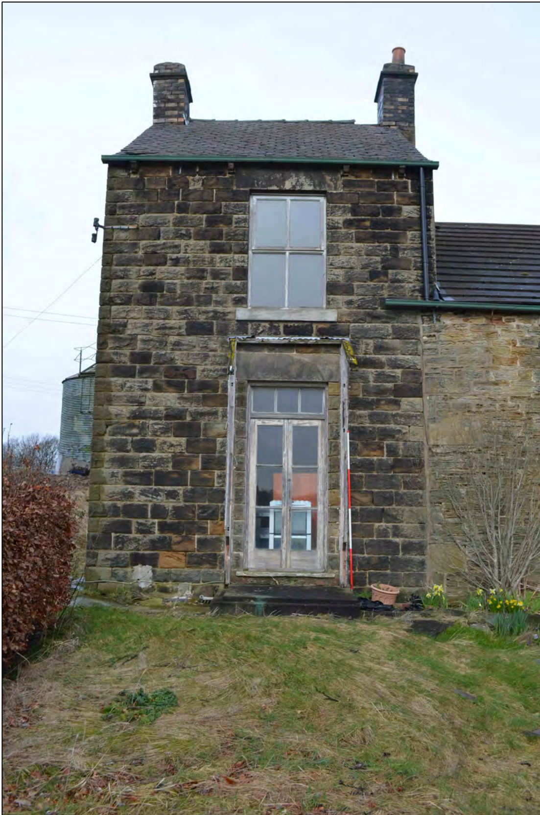
Appendix 2.28: View of Building 2, looking north
