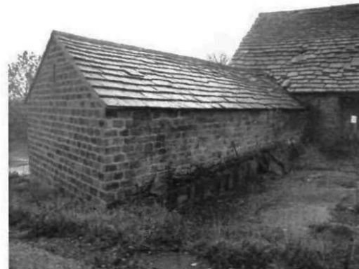
Fig 10 Single storey building – south east corner – Barn B
