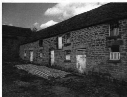
Fig 7 West elevation – Barn B
