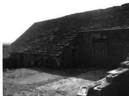
Fig 9 East elevation – Barn B
