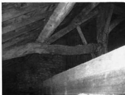
Fig 14 Half truss from timber post
