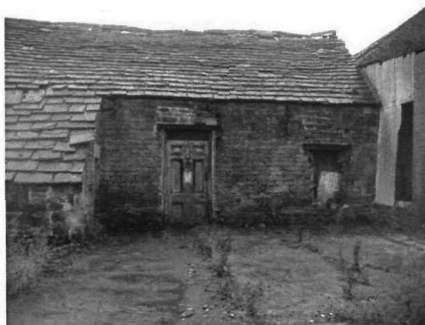
Fig 17 East elevation – Barn B – north end
