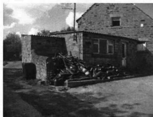
Fig 8 Outbuilding to south of Barn B
