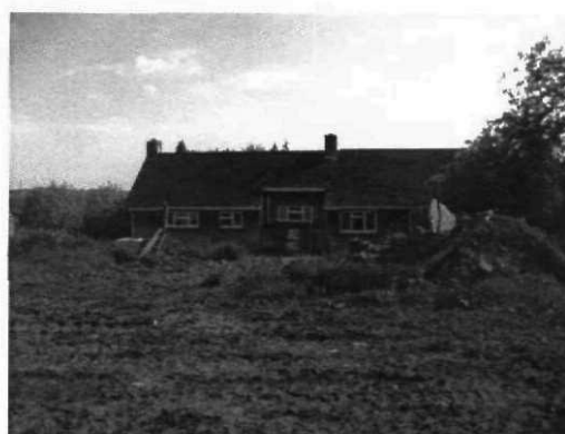
Fig 2 North elevation of bungalow
