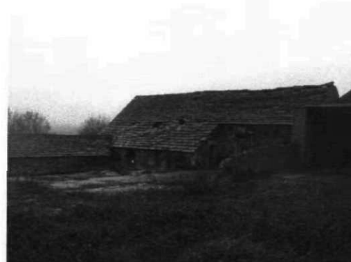
Fig 12 North and east elevation – Barn B
