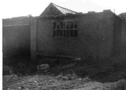
Fig 6 Brick extension to NE corner - Barn A
