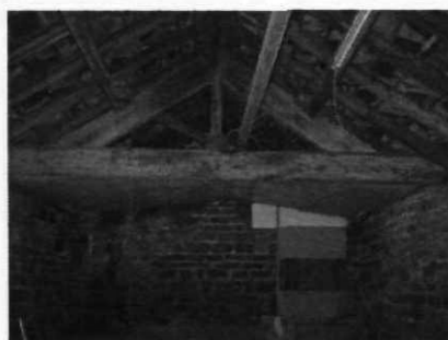
Fig 19 End truss looking west
