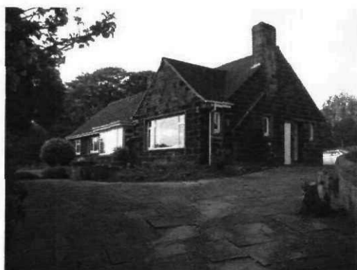
Fig 1 South and east elevation of bungalow
