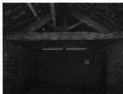
Fig 20 End truss looking east
