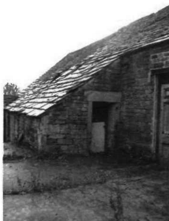
Fig 11 Rear catslide – Barn B
