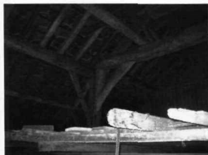
Fig 13 Barn A roof structure
