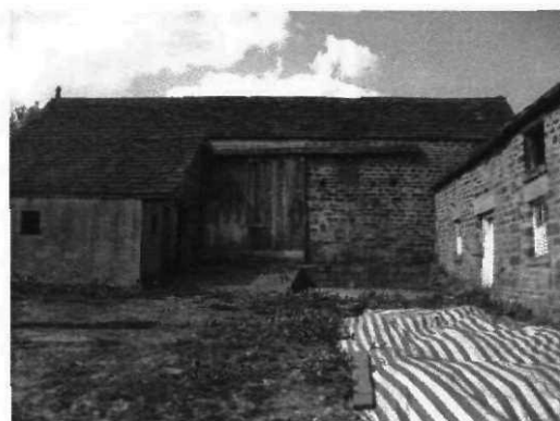
Fig 3 South elevation – Barn A
