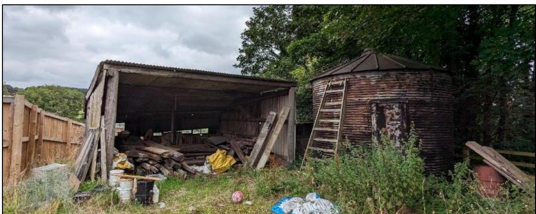
Plate A6.13. Building G
