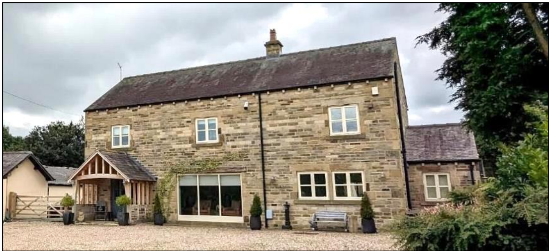
Plate A6.12. Building F
